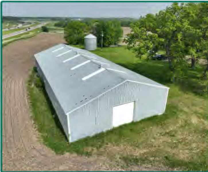
West view of Shed
