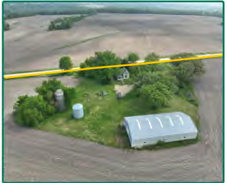
View of Building Site
