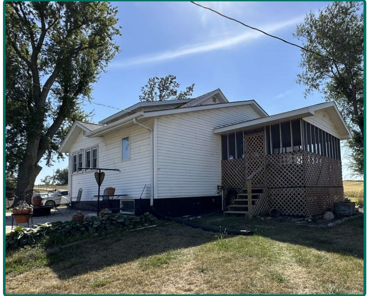
House—North and East Sides
