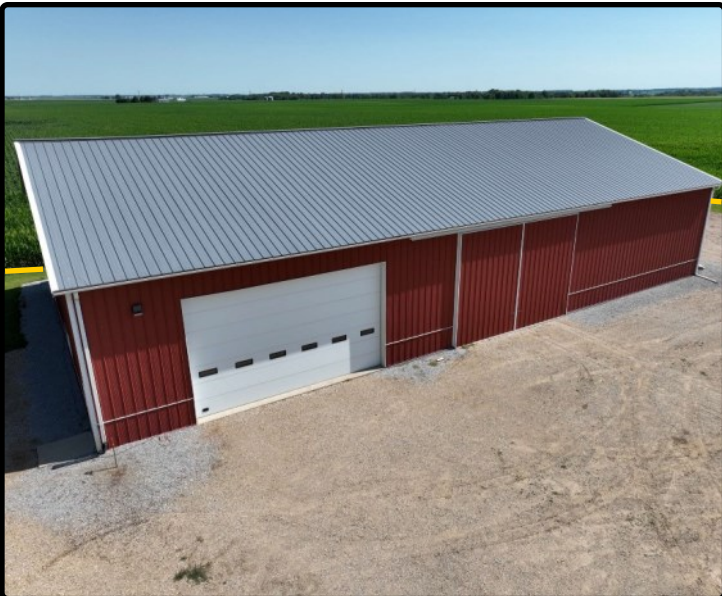
Parcel 4 - Pole Building
