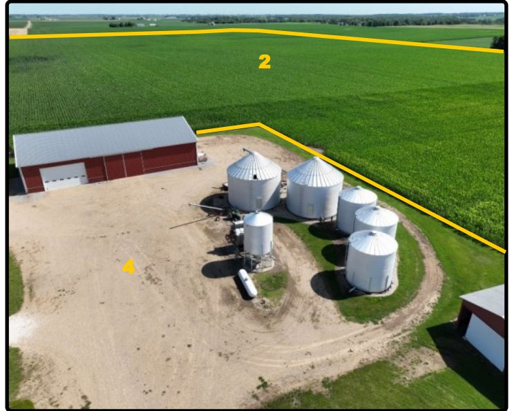
Parcel 4 - Pole Building & Grain Storage
