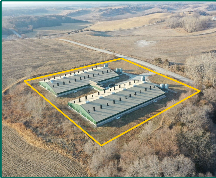
West Site - Looking Northwest
