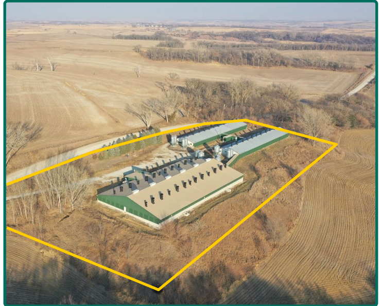
East Site - Looking Northeast
