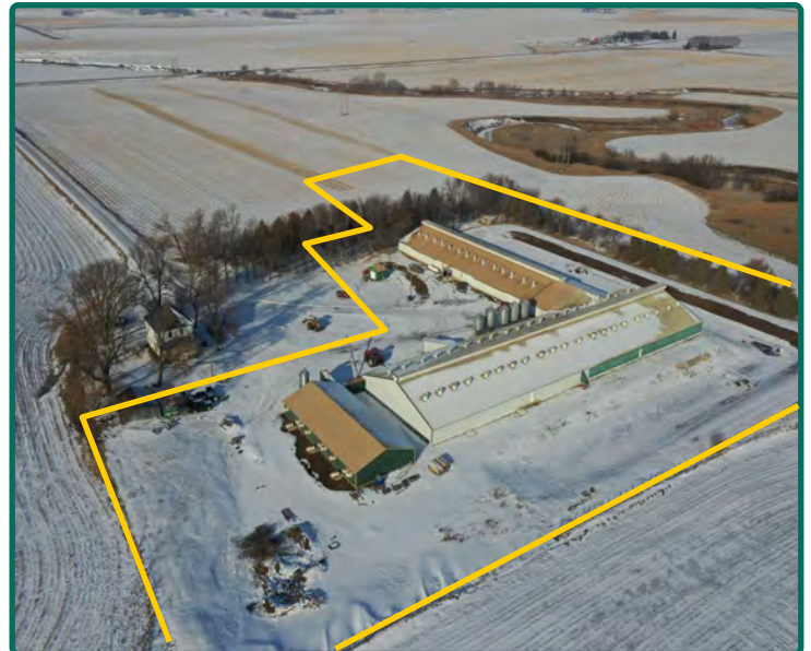
Southeast looking Northwest
