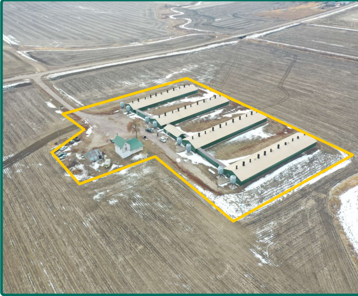
Northeast looking Southwest
