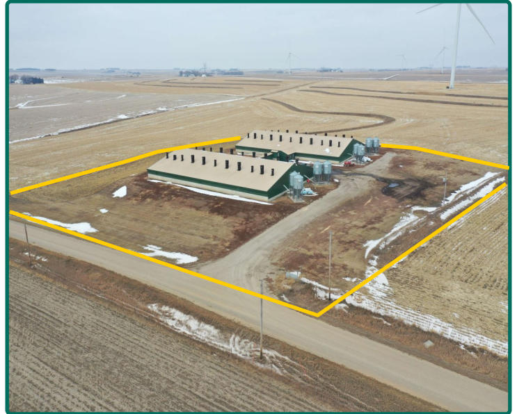
Southeast looking Northwest
