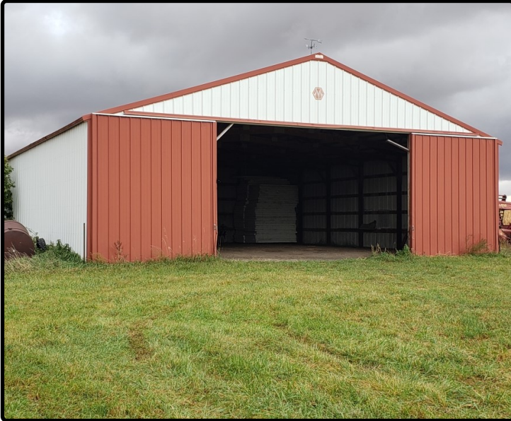
Parcel 2 - 54' x 48' Machine Shed
