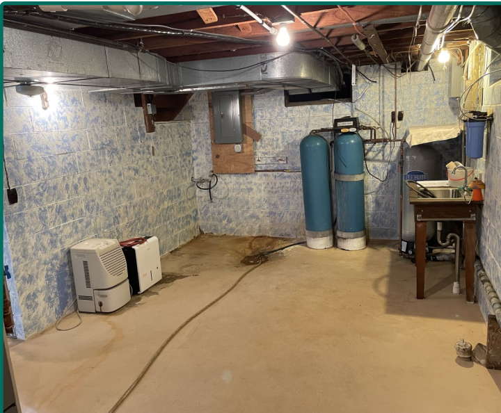
New Electrical System in 2021
