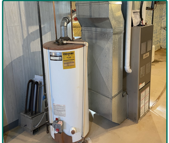
Furnace & Water Heater
