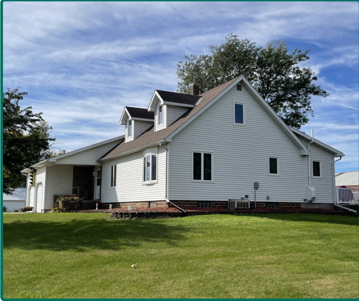
Northeast Corner of House
