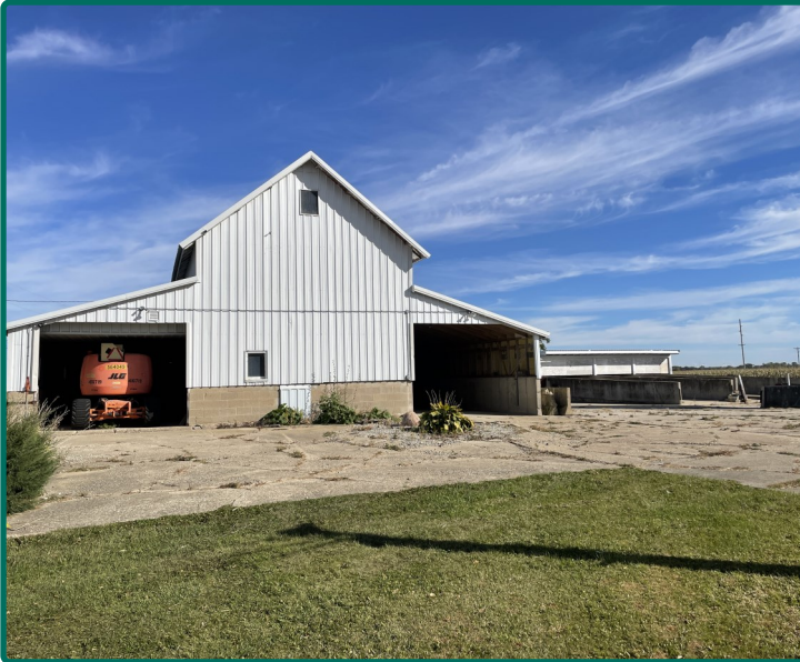
South Side of Barn & Lean-Tos
