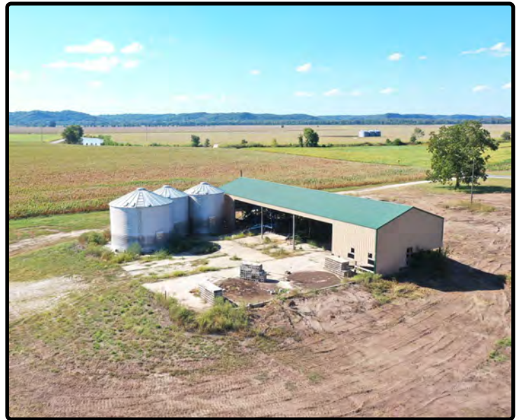
Parcel 4 - Bins and Machine Shed
