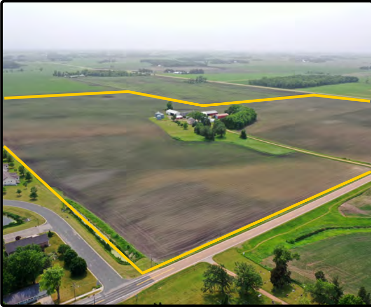
Northeast corner looking Southwest
