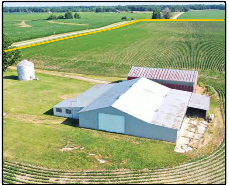
Parcel 3 - Bin and outbuildings
