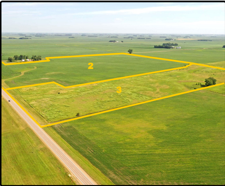
Parcels 2 & 3 - Looking North
