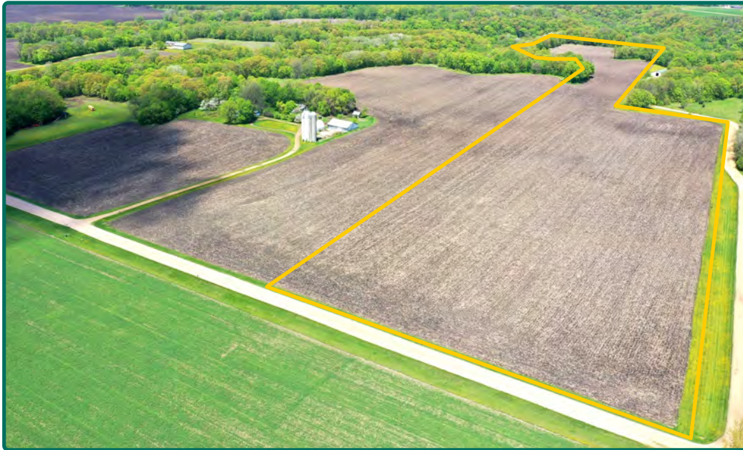
Southeast Looking Northwest
