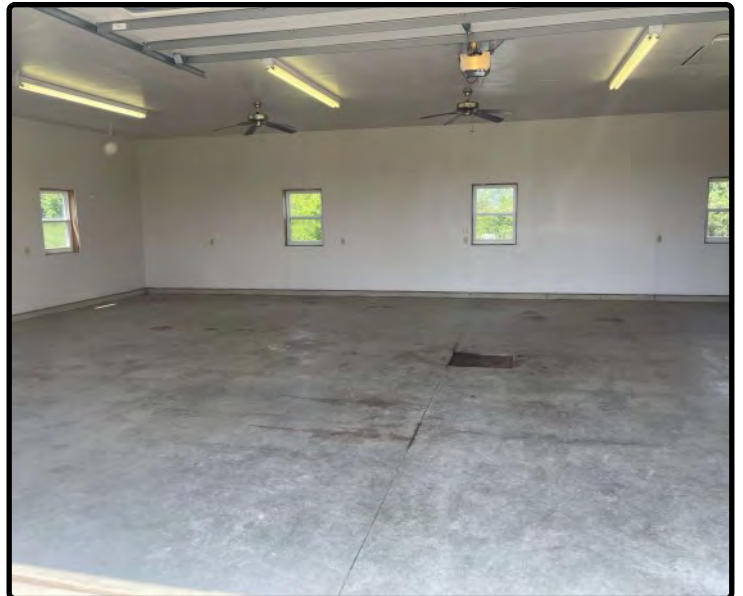
Parcel 2 - Garage With In-floor Heating
