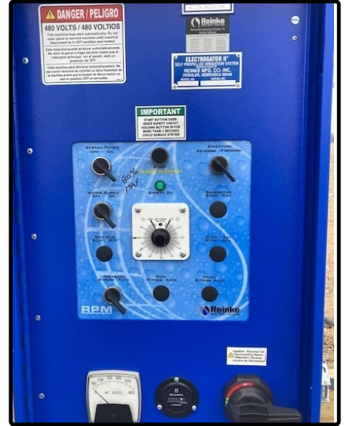
Panel 2 on North Tower
