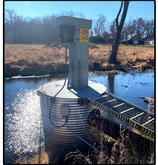
West Lift Pump
