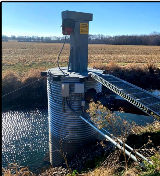
East Lift Pump
