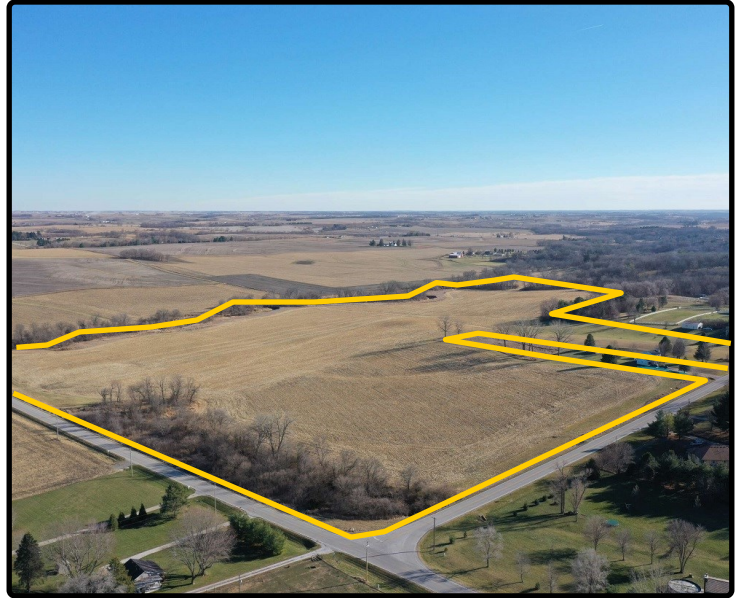
Northwest Looking Southeast
