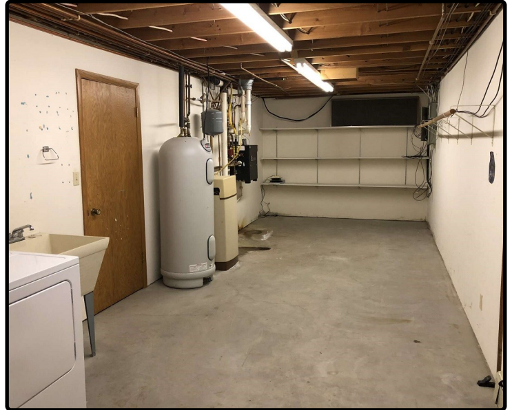
Basement Utility Room
