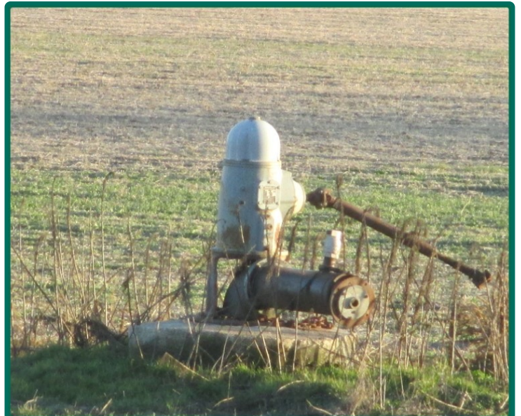
2nd Well along West Side of Property
