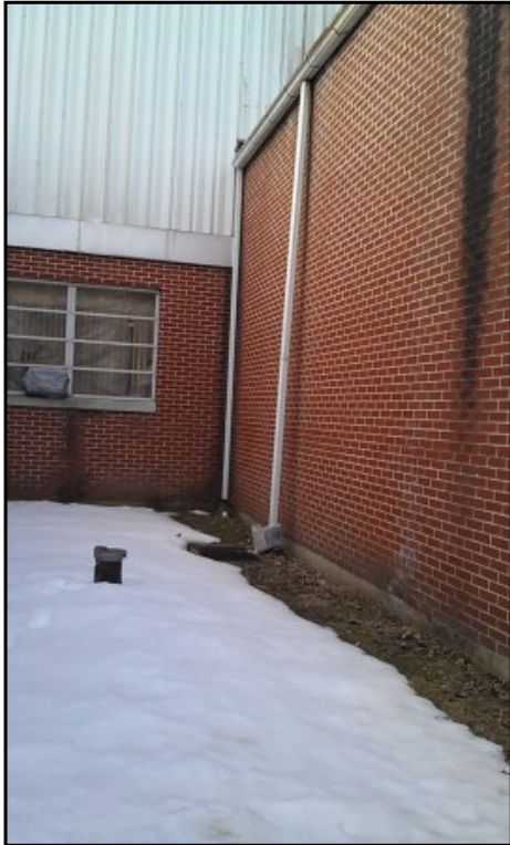
WELL AND DRAINPIPE DRAINAGE
