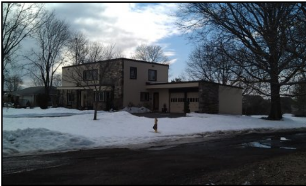
SIDE NEIGHBOR SW
