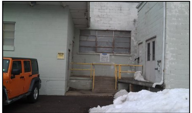
SW SIDE CONTINUING TO REAR
