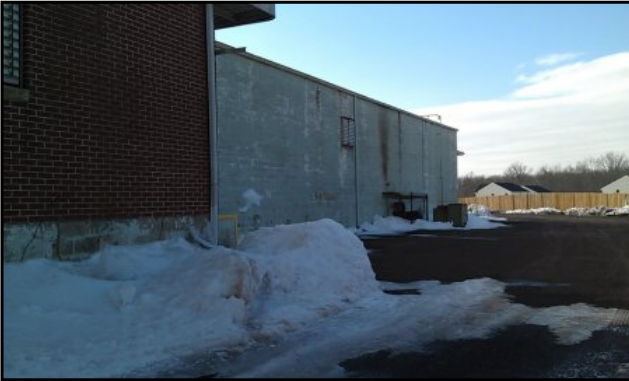
NORTH SIDE CONTINUING TO REAR
