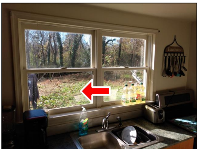
4.6 Item 3(Picture) Both inoperable. Left side broken thermal seal.
