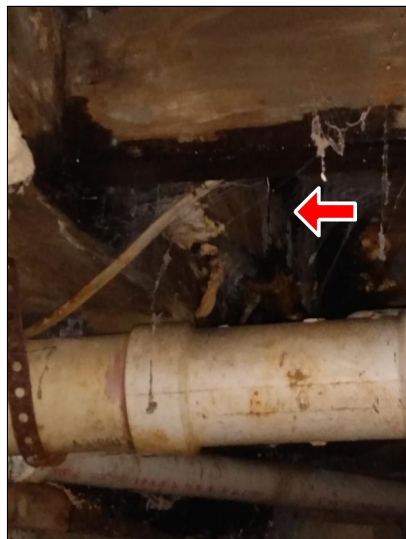
6.0 Item 2(Picture) Wet with dark staining.
