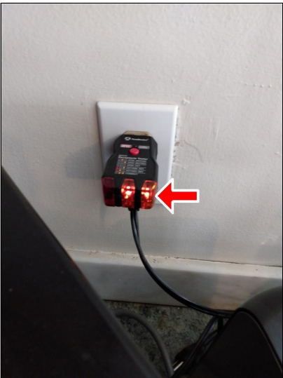
7.5 Item 2(Picture) Not GFCI protected.
