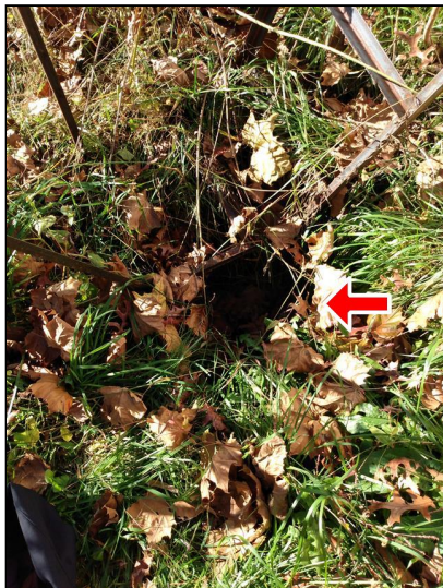
2.4 Item 4(Picture) Deep hole.
