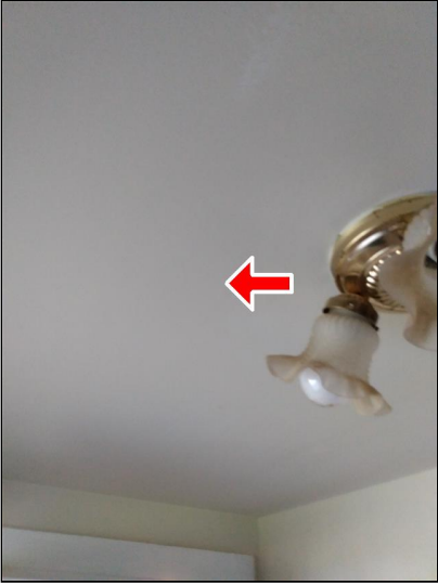
9.4 Item 3(Picture) No exhaust fan.
