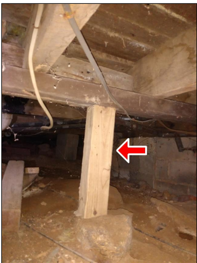
5.3 Item 5(Picture) A wooden pier, not plumb.
