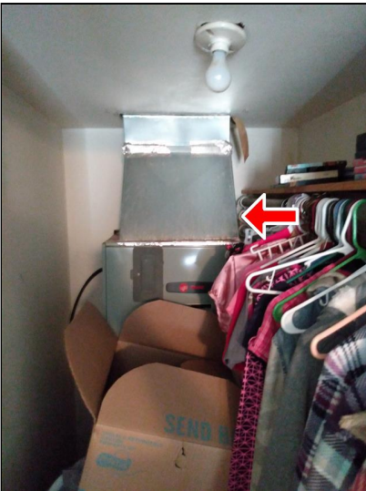
8.0 Item 3(Picture) Air handler.
