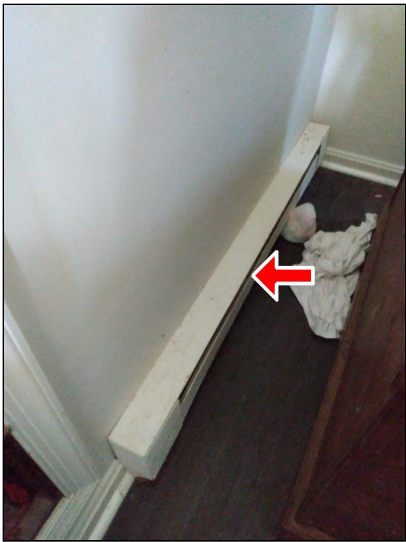
8.0 Item 6(Picture) Inoperable.
