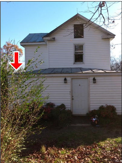
5.5 Item 1(Picture) Sagging.
