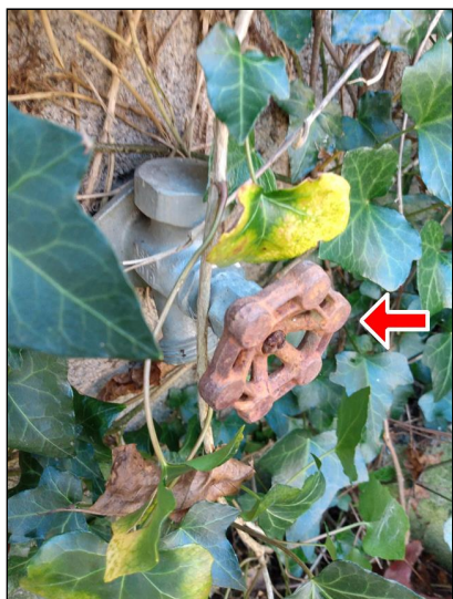
6.1 Item 1(Picture) Did not deliver water.
