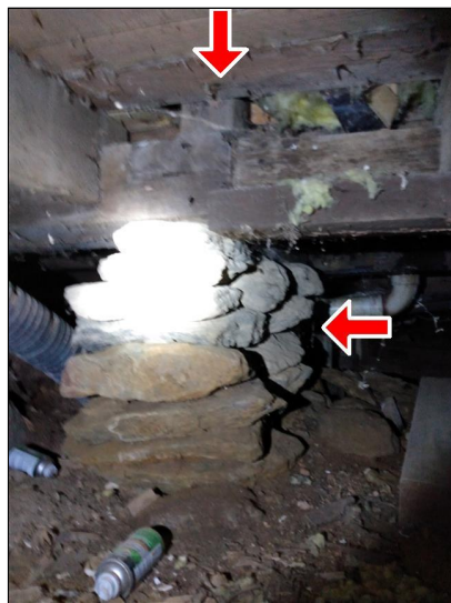
5.3 Item 6(Picture) Dry stacked stone with repair above.
