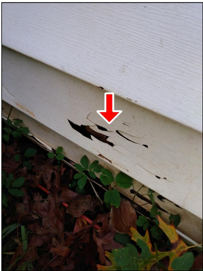
2.0 Item 5(Picture) Broken.
