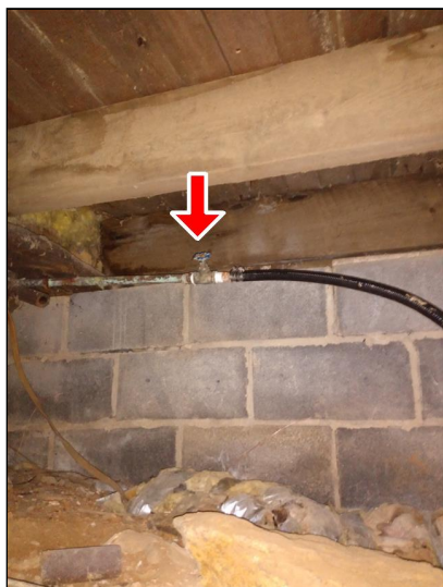
6.3 Item 1(Picture) Main water shut off.
