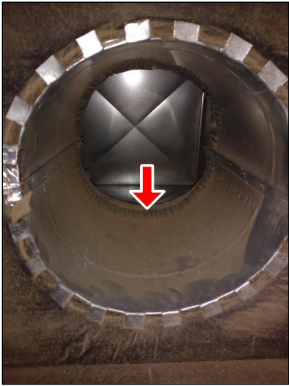
8.3 Item 2(Picture) Dirty.
