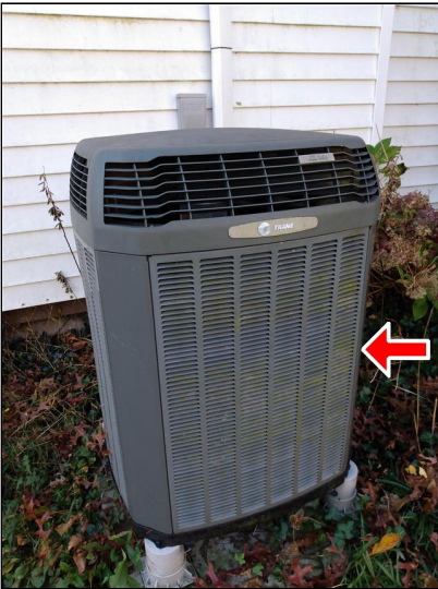
8.0 Item 1(Picture) Heat pump.
