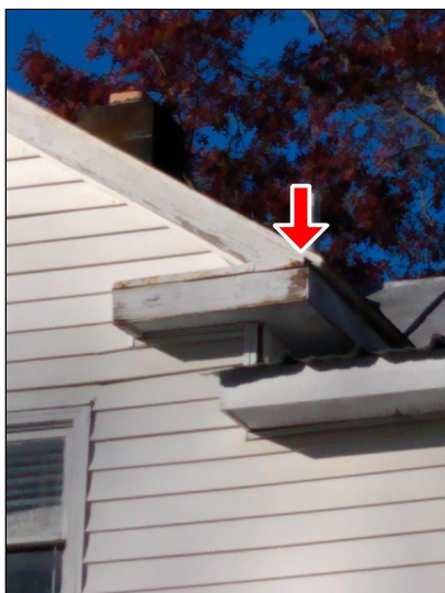
2.5 Item 1(Picture) Moisture damage.
