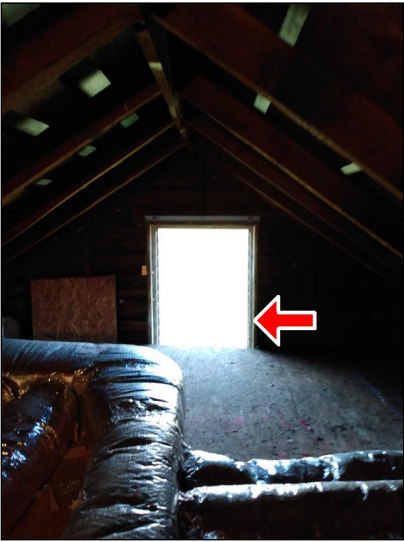
4.6 Item 4(Picture) Inoperable.
