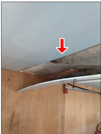
3.0 Item 1(Picture) Falling.
