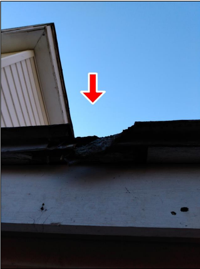
1.0 Item 1(Picture) Example of damaged roofing.
