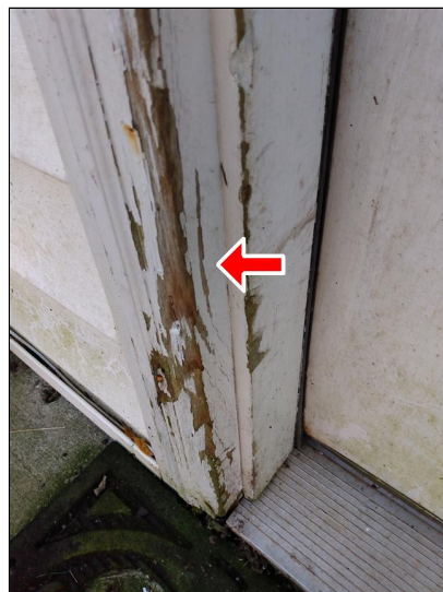
2.0 Item 2(Picture) Flaking/missing paint.
