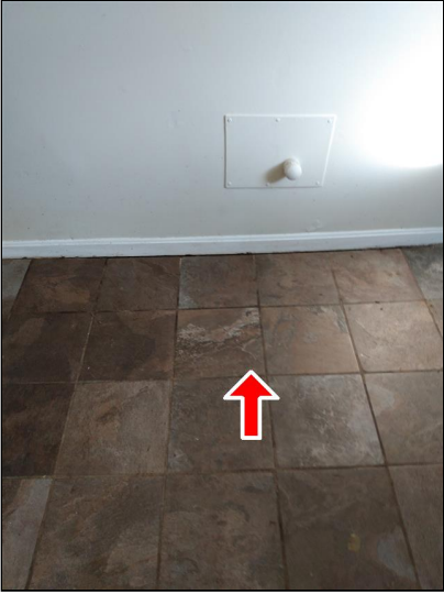
4.2 Item 1(Picture) Example of wavy flooring.
