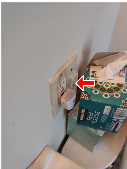
7.6 Item 2(Picture) Odd GFCI operation.
