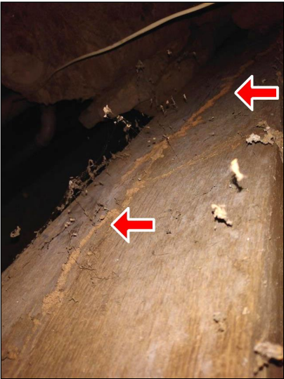
5.3 Item 7(Picture) Mud tubes.
