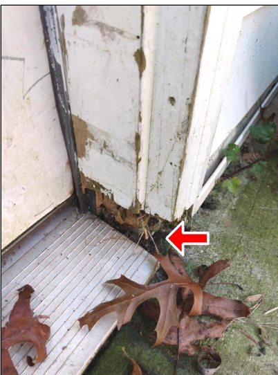
2.0 Item 1(Picture) Moisture damage.
