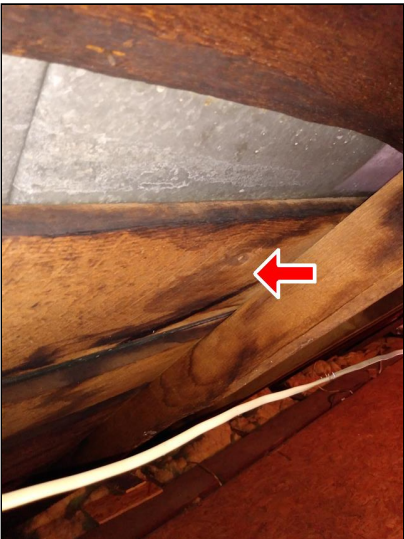
5.5 Item 3(Picture) Example of dark staining.
