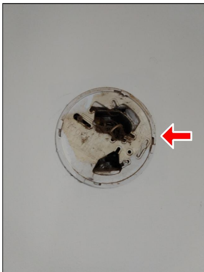
7.8 Item 1(Picture) Missing.
