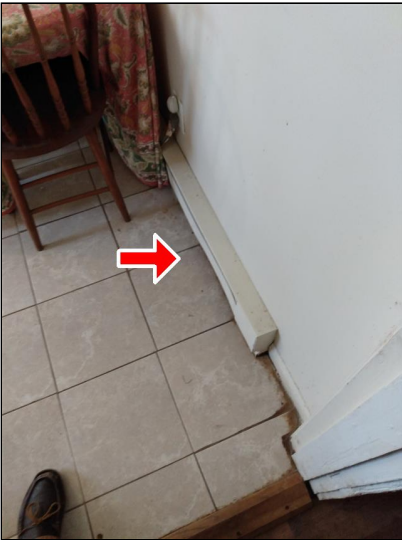
8.0 Item 7(Picture) Kitchen's electric baseboard heat.
