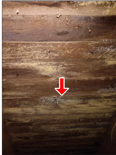
5.3 Item 4(Picture) Example of the fuzzy substances.
