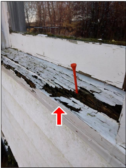
2.2 Item 1(Picture) Example of moisture damage.
