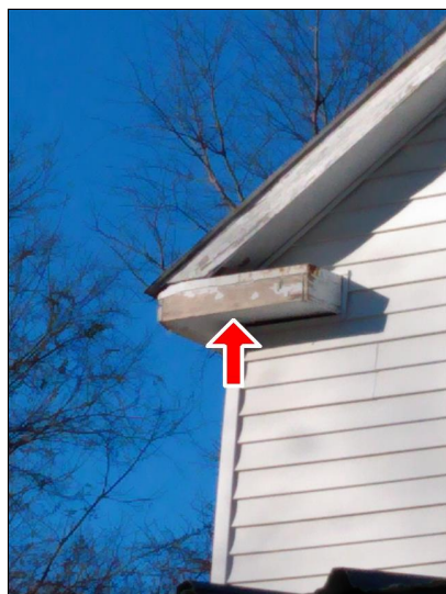
2.5 Item 2(Picture) Peeling paint, separated materials.
