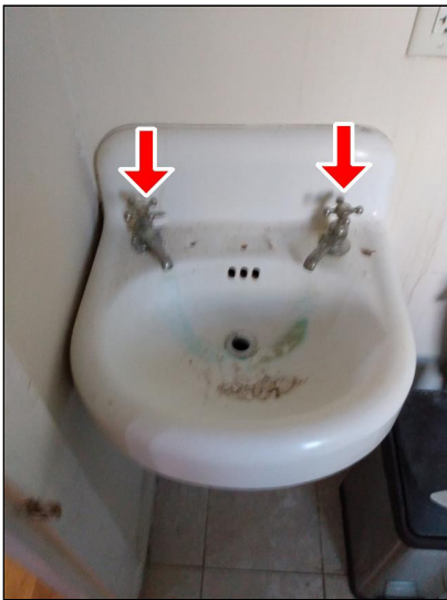
6.1 Item 2(Picture) Did not deliver water.
