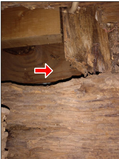
5.3 Item 1(Picture) Example of dry rot.
