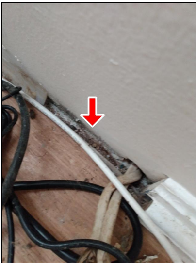
4.2 Item 4(Picture) Example of missing molding & gaps between floors & walls.
