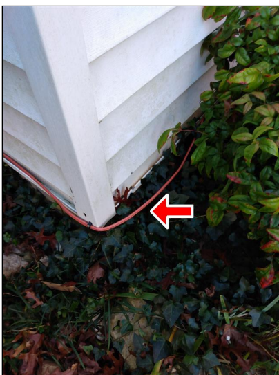
7.4 Item 1(Picture) Heat pump wiring.
