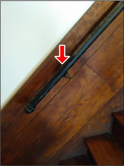
4.3 Item 2(Picture) Here.
