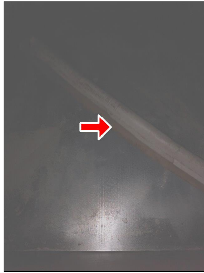
8.3 Item 3(Picture) Debris in ducting.
