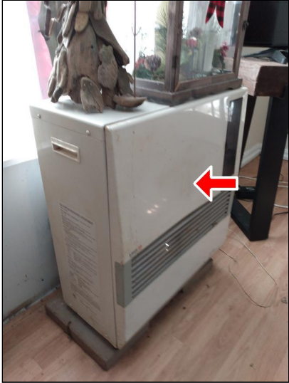
8.0 Item 4(Picture) Not tested.
