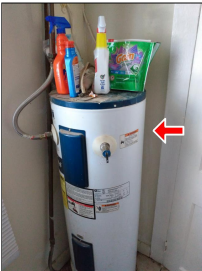
6.2 Item 1(Picture) Water heater.
