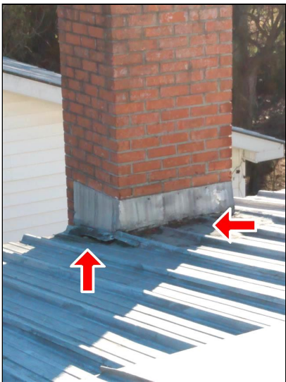
1.1 Item 2(Picture) Example of flashing pulling up and tar repairs.
