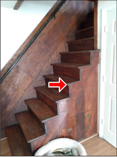
4.3 Item 1(Picture) No railing.
