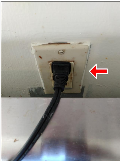
7.6 Item 1(Picture) Not GFCI protected.
