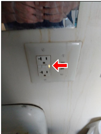
7.6 Item 3(Picture) Did not reset to re-energize.
