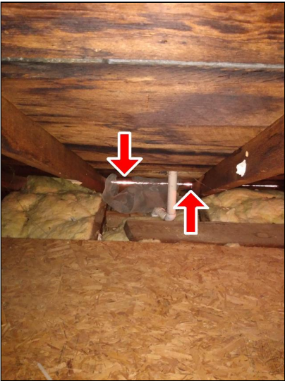
5.5 Item 2(Picture) Daylight.
