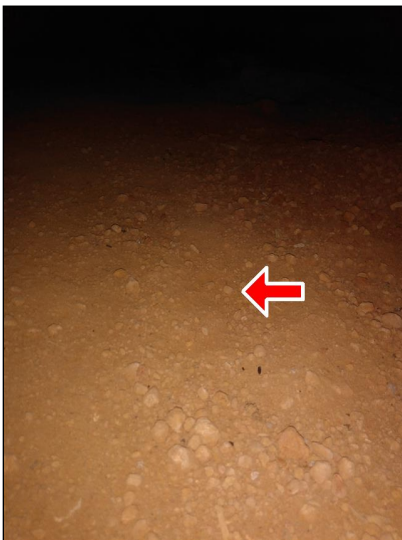
9.2 Item 1(Picture) Bare crawsapce soil.
