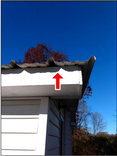
1.1 Item 1(Picture) Example of an area with no flashing.
