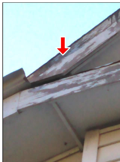
2.5 Item 3(Picture) Peeling paint, separated materials.
