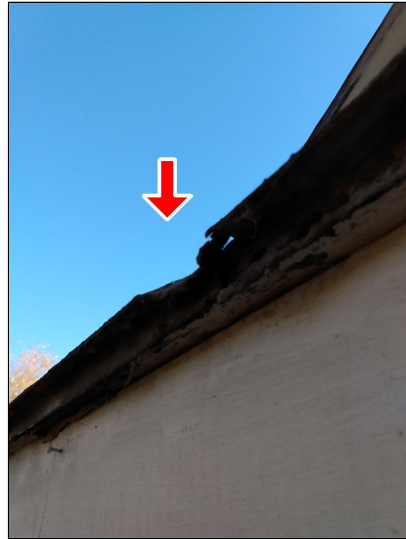
1.0 Item 2(Picture) Example of damaged roofing.
