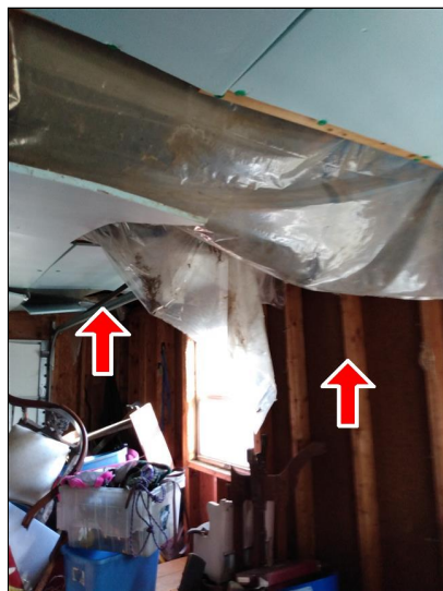
3.0 Item 2(Picture) Falling.
