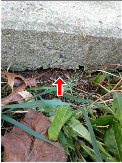
2.4 Item 1(Picture) Example of Undermining.
