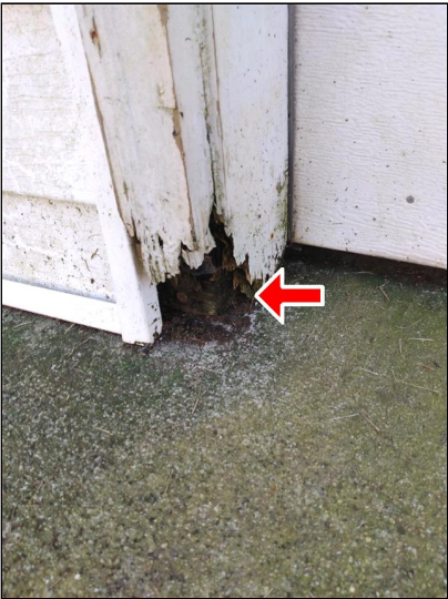
3.4 Item 2(Picture) Moisture damage.
