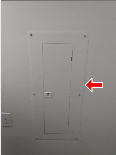
7.0 Item 1(Picture) Main distribution panel.
