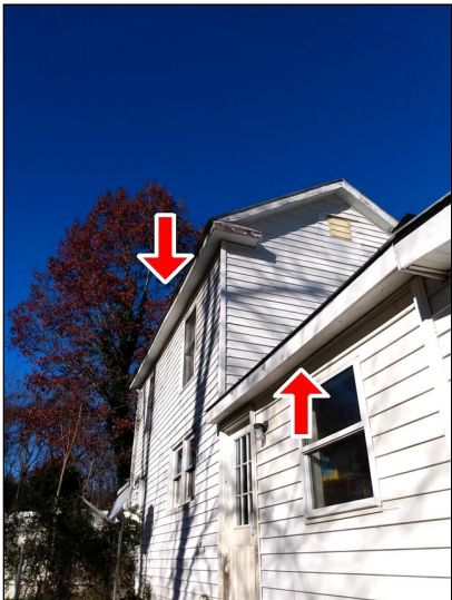
1.3 Item 1(Picture) No gutters.
