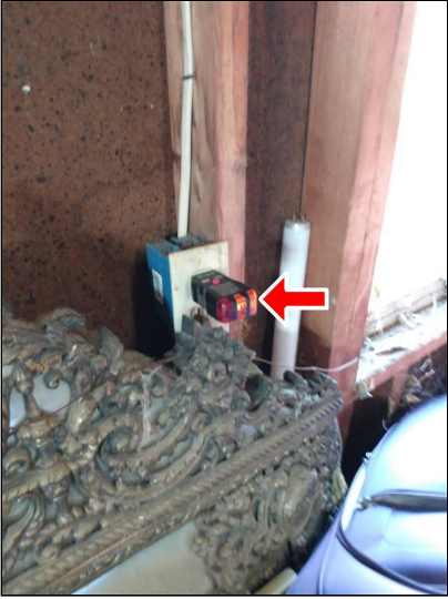
7.5 Item 1(Picture) Not GFCI protected.
