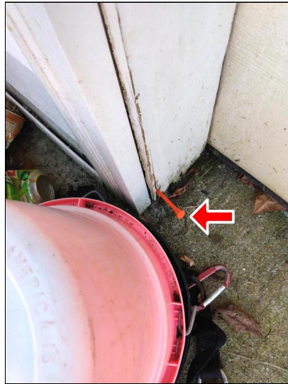
3.4 Item 3(Picture) Moisture damage.
