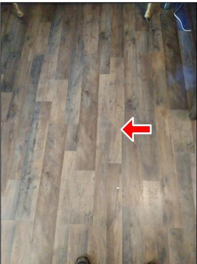
4.2 Item 3(Picture) Flooring is popped up.
