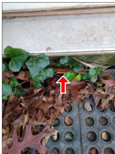
7.4 Item 2(Picture) Heat pump wiring.
