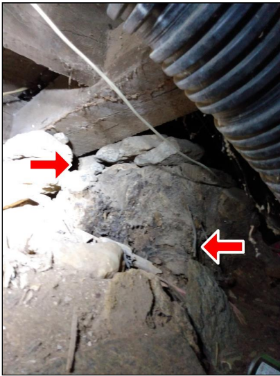
5.2 Item 1(Picture) Stump & dry stacked stone.
