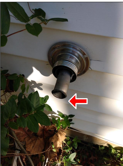
8.5 Item 1(Picture) No cap or heat shield.
