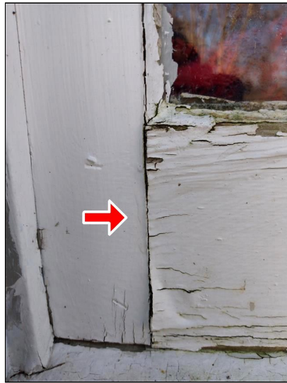
2.2 Item 2(Picture) Example of moisture damage.
