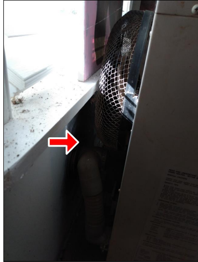
8.0 Item 5(Picture) In contact with combustibles.
