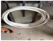
#30D • 3/4 inch Pex water line
