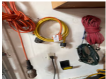
#149 • Extension cords and drop light
