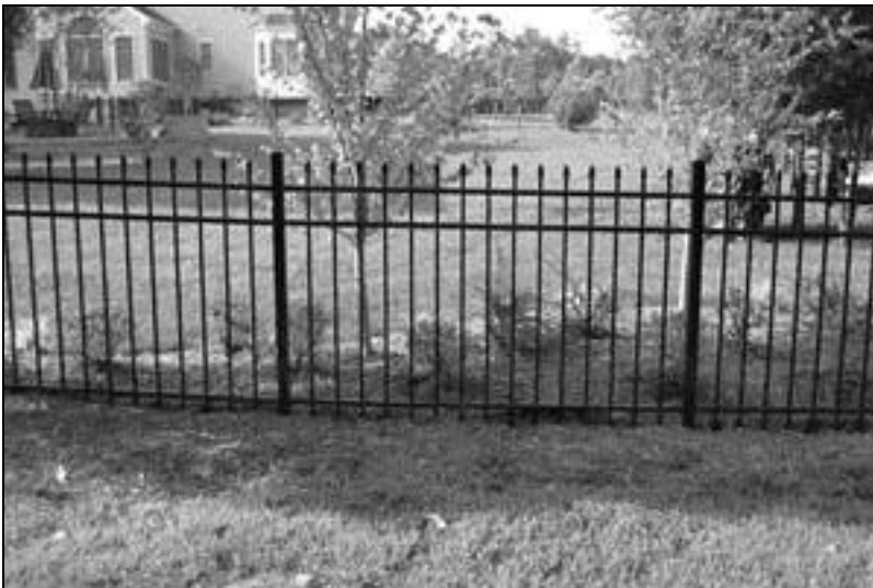
Figure A1-1: Four foot black aluminum fence with spikes on top.
