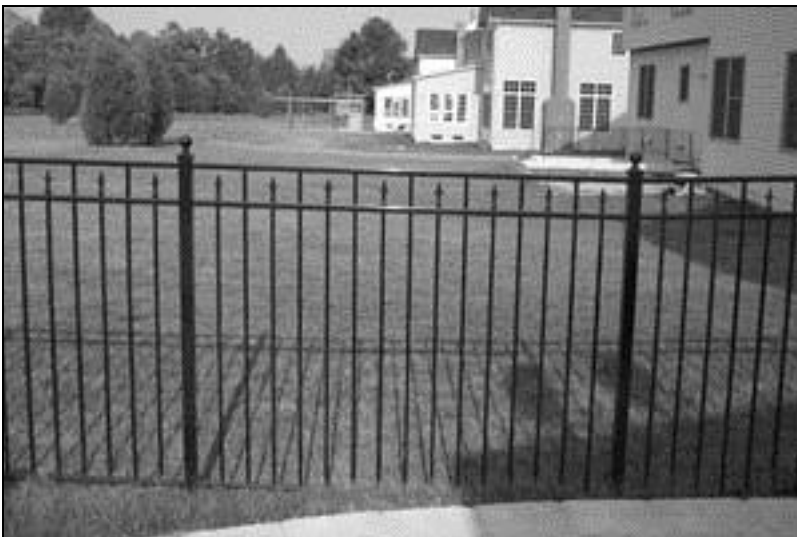
Figure A1-2: 5-foot black aluminum fence, with spikes and a floating safety bar across the top.
