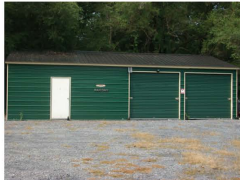
Lot 1 Metal building : 40' x 24' 2- 8x8 roll up doors & 1 personnel door
