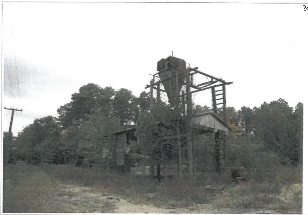
Photograph No. 24 Mill structure east of main building, view to the northeast.
