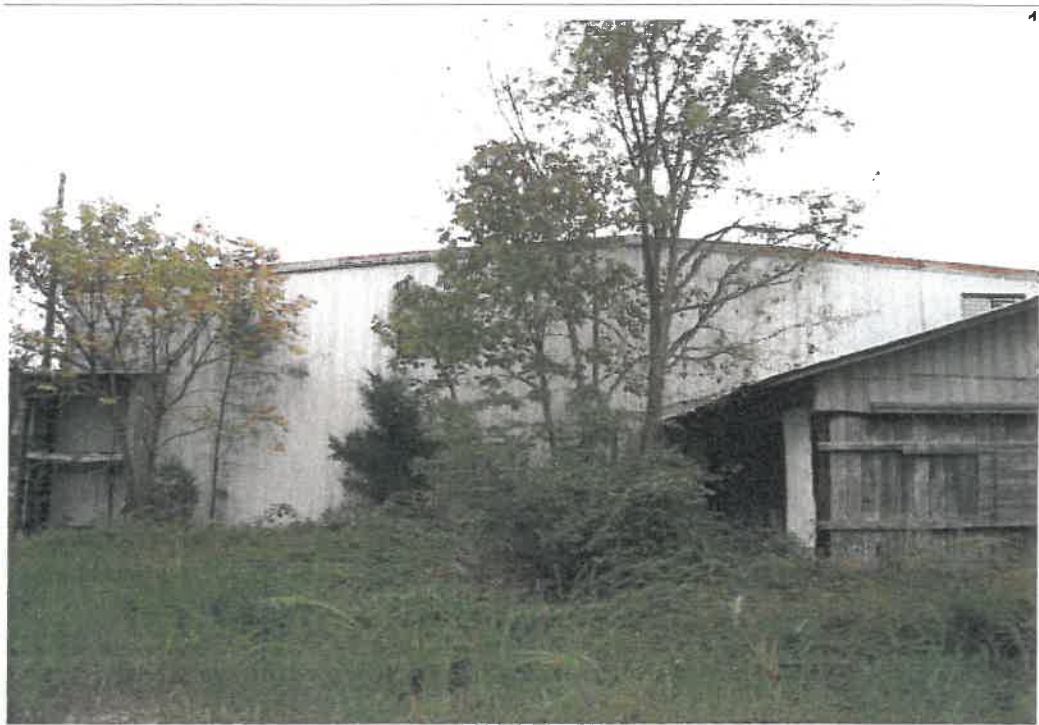
Photograph No. 13 Main building north elevation, view to the south
