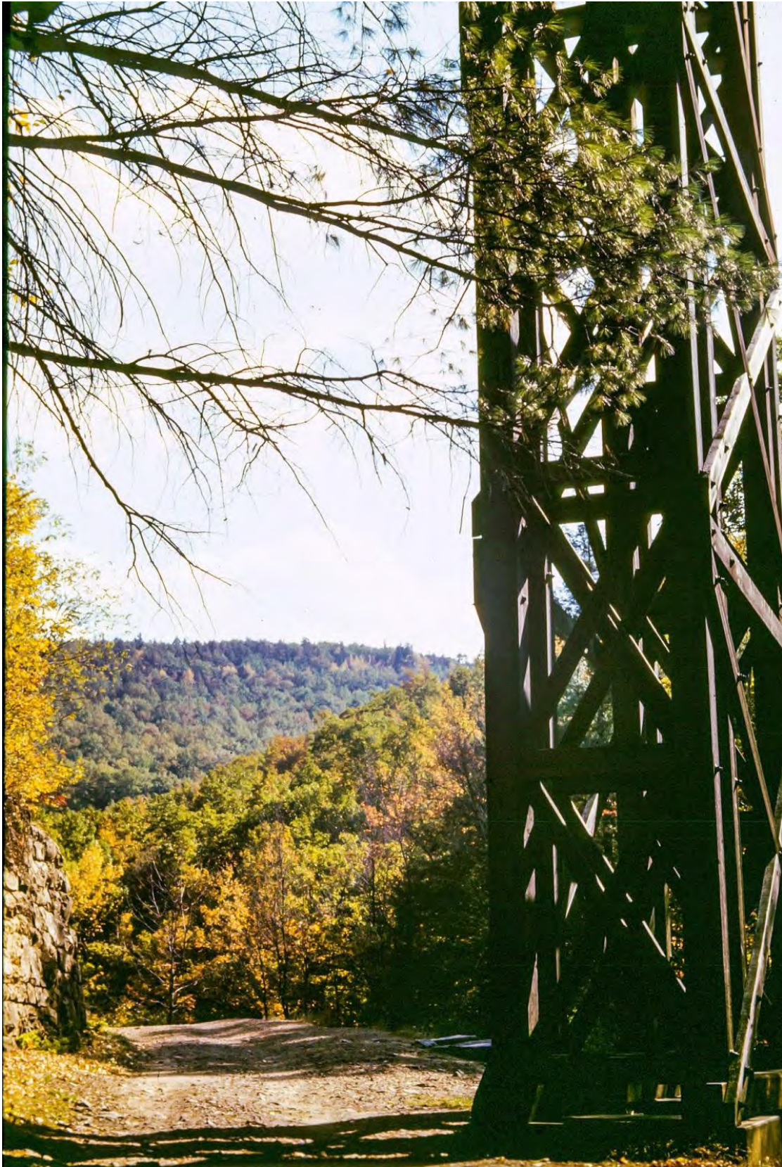
Under Highbridge, looking South, the above road went Northeast, past "The Deep Hole" and into the "Jeff Swamp" area. According to local lore, the two wooden Highbridge supports were erected during World War One to support heavier RR engines and heavier freight cars; the above support was at the East end of the bridge.
