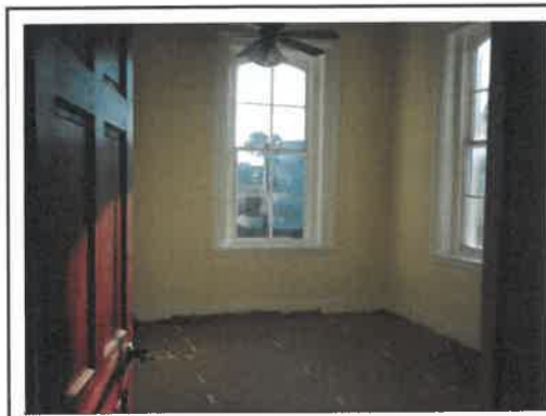
Subject Property Interior Finish, 2 nd Floor
