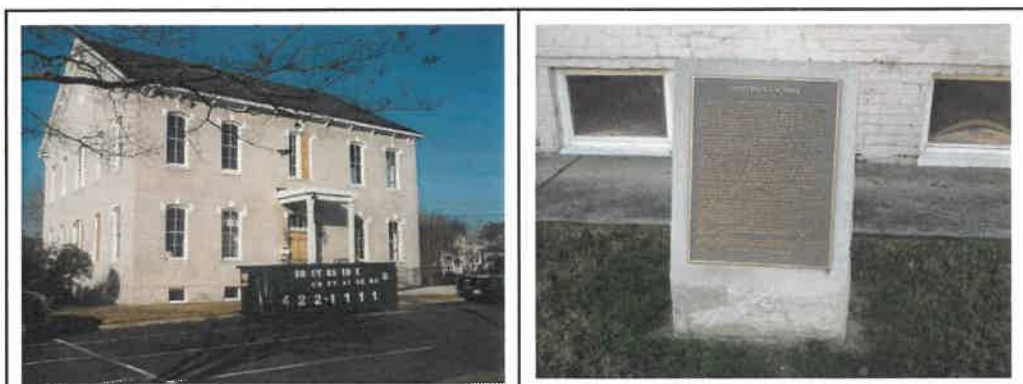
Subject Property Rear (East) Elevation
