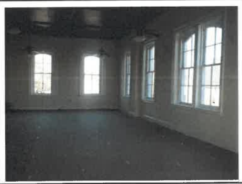
Subject Property Interior Finish, 2 nd Floor
