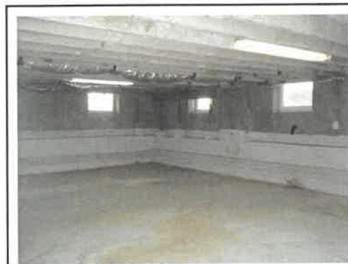
Subject Property Interior Finish, Basement
