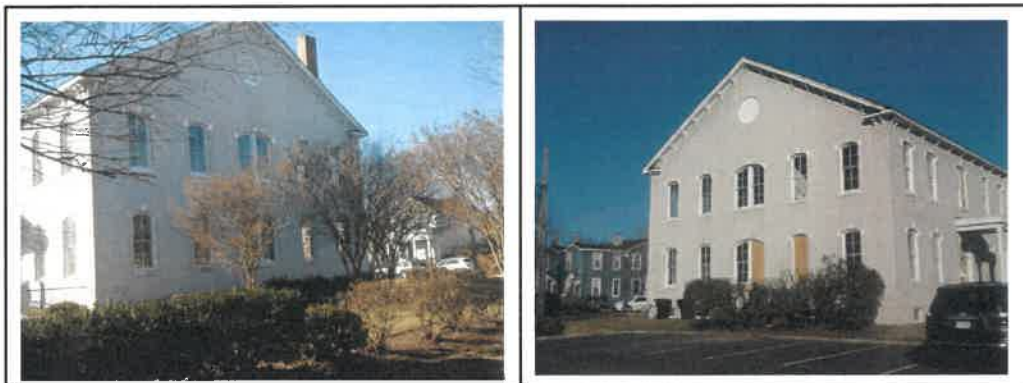
Subject Property Side (North) Elevation
