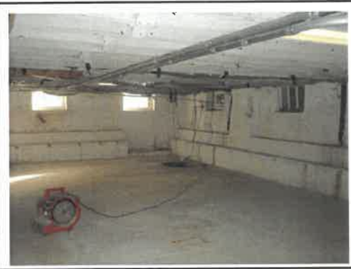
Subject Property Interior Finish, Basement
