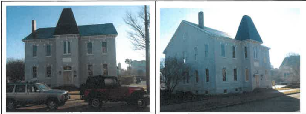
Subject Property Front (West) Elevation
