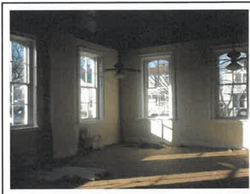
Subject Property Interior Finish, 1 st Floor
