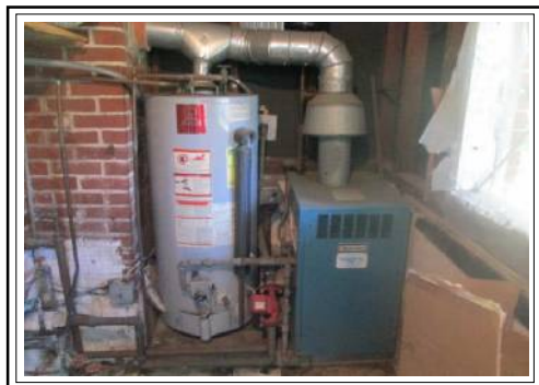
WATER HEATER & NATURAL GAS BOILER
