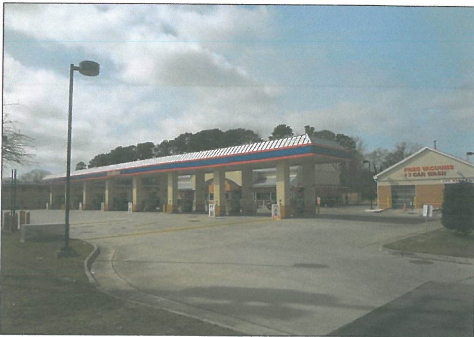
SUBJECT PROPERTY PHOTOGRAPH TAKEN ON MARCH 29, 2018. (Additional photographs of the subject property are included in the Physical Description.)
