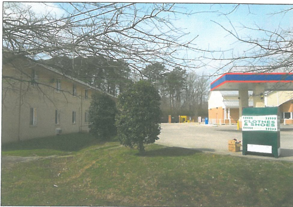
PHOTOGRAPH TAKEN ALONG THE SOUTH PROPERTY LINE.
