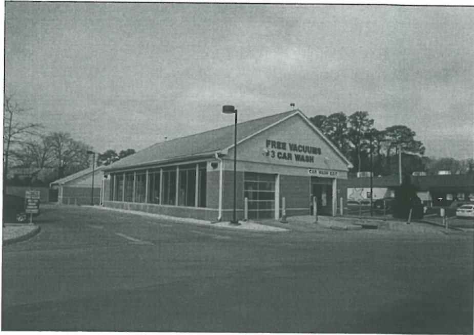
VIEW OF THE CAR WASH AND AUXILIARY BUILDING.
