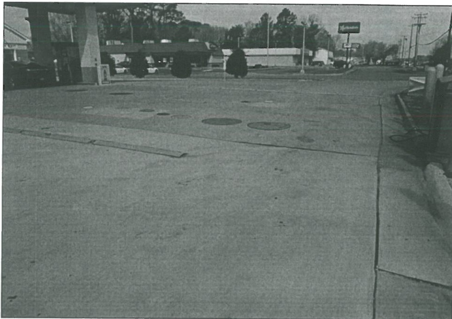
VIEW OF THE TANK FIELD.
