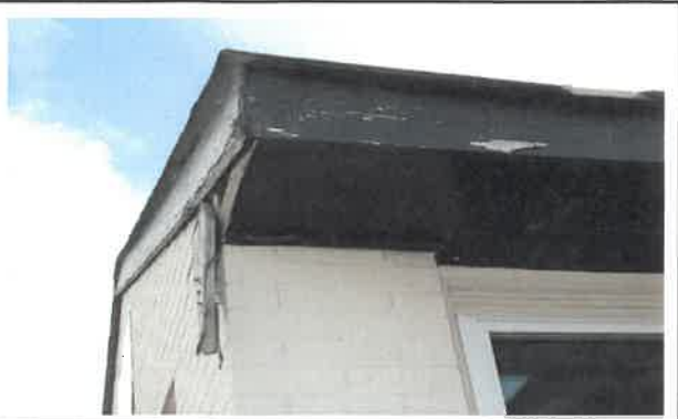
Damaged Trim Boards
