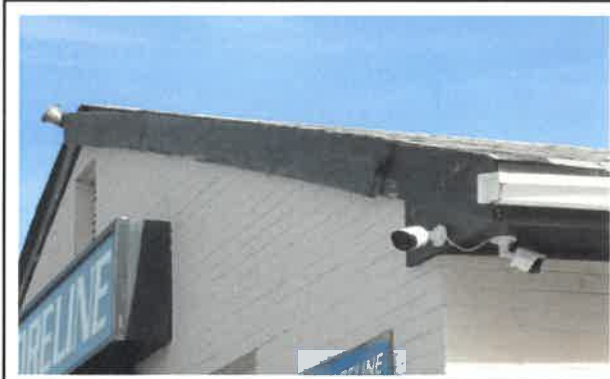
Damaged Trim Boards and Gutter
