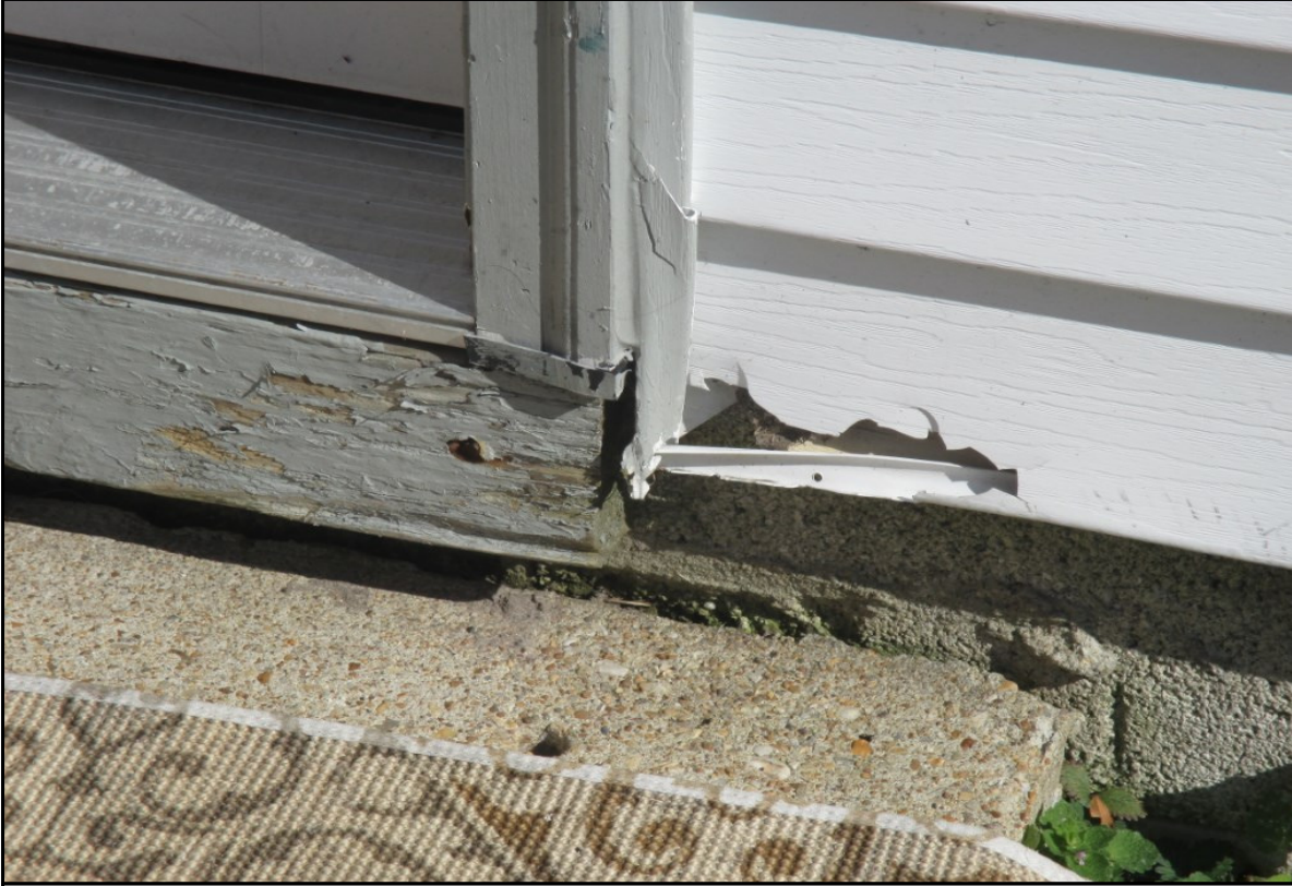
Broken siding right side
