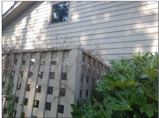
4.11.A HEATING & COOLING Photo 1
