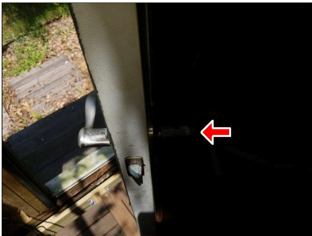
2.2(6) ENTRY DOORS Photo 2
