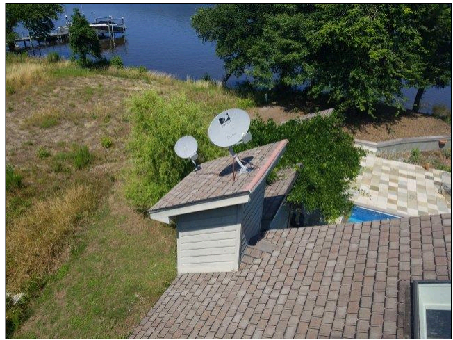
1.2 CHIMNEY / VENT #1 Photo 1
