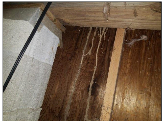
9.2(1) FLOOR FRAMING Photo 2
