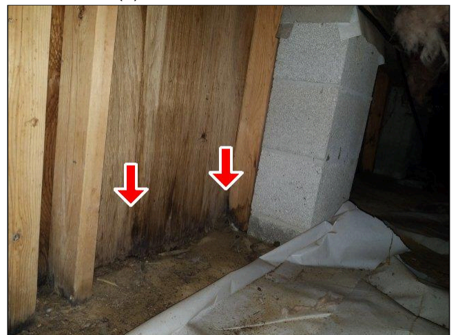
9.2(2) FLOOR FRAMING Photo 1
