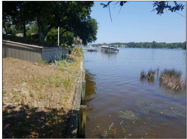
3.5 BULKHEAD / DOCK Photo 2
