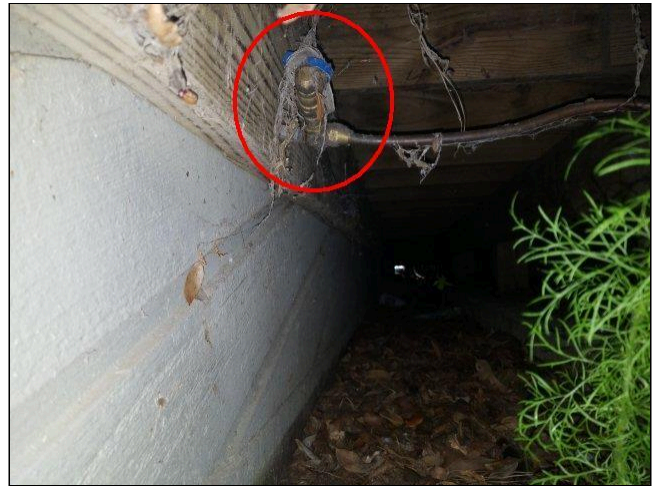
8.10(1) FIREPLACE GAS BURNERS Photo 2
