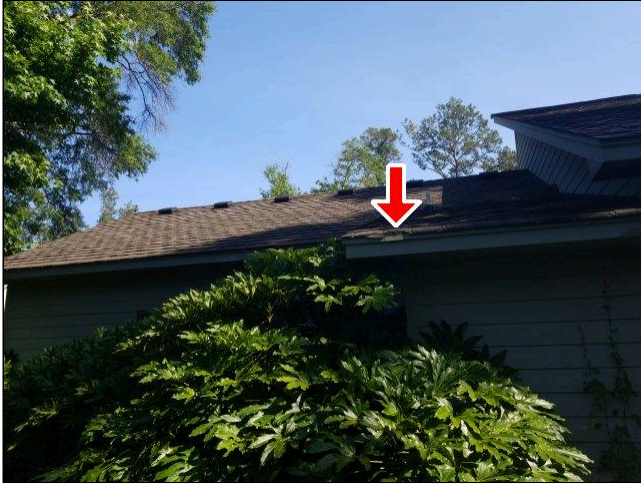
4.0.A ROOFING Photo 1
