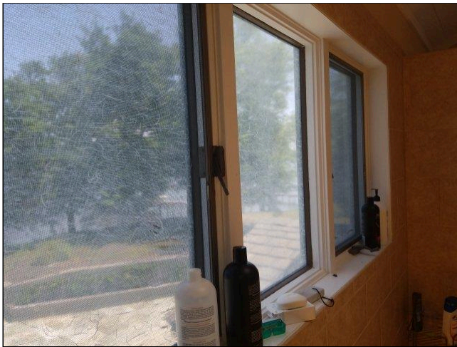
6.6.C(3) WALLS / CEILINGS Photo 1
