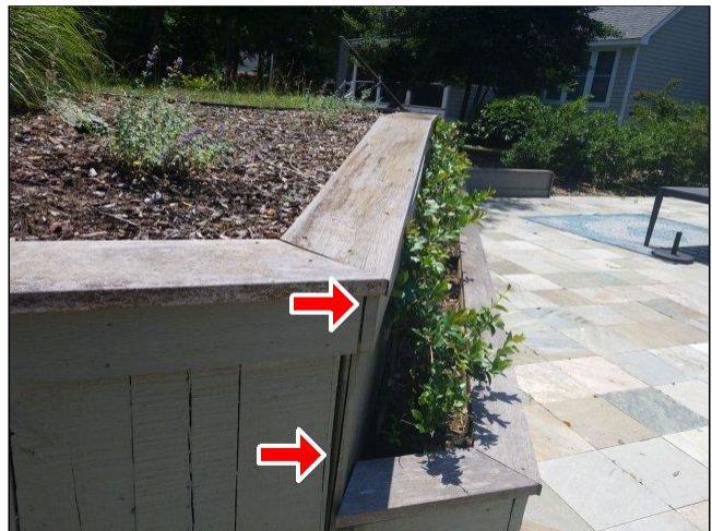
3.2 RETAINING WALL(S) Photo 3
