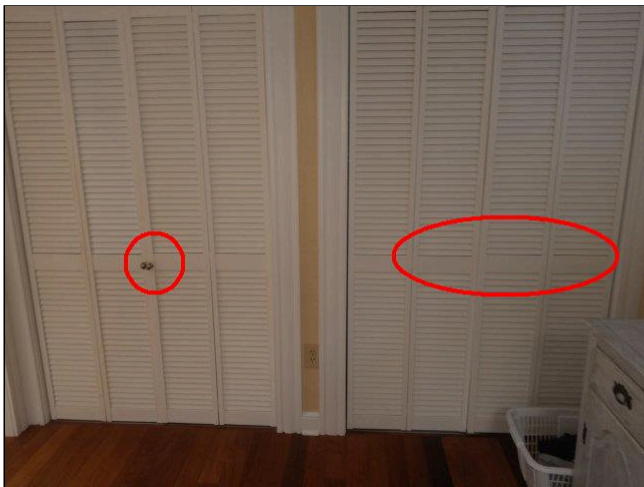
8.7(3) ROOM DOORS Photo 1
