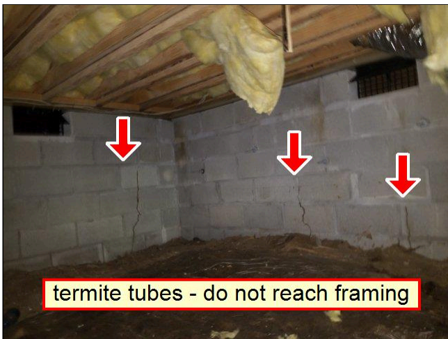
9.2(1) FLOOR FRAMING Photo 1
