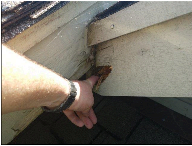
1.9 FASCIA / SOFFITS Photo 1
