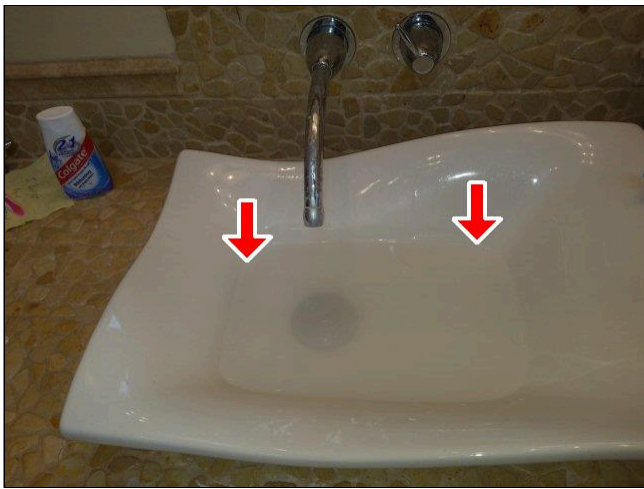
6.0.C SINK(S) Photo 1
