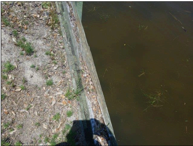
3.5 BULKHEAD / DOCK Photo 3
