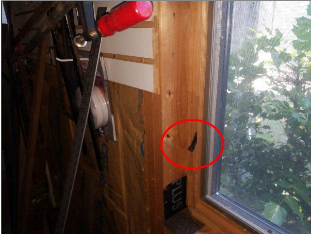
4.5.A WINDOWS Photo 1
