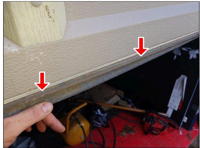
4.8.A OVERHEAD/VEHICLE DOOR(S) Photo 1
