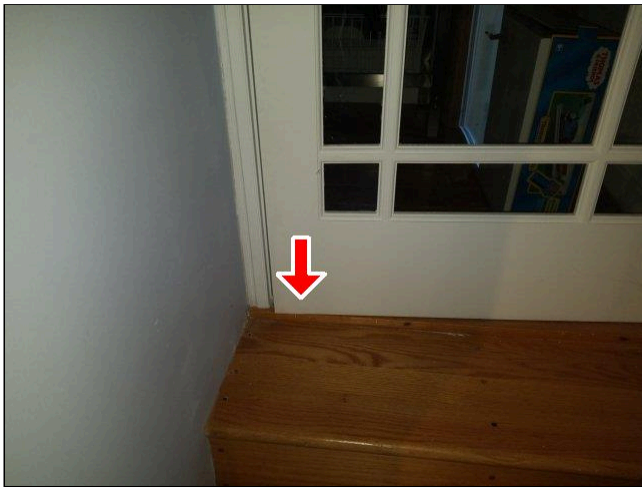
4.4.B(2) WALLS / CEILINGS Photo 1
