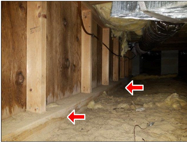
9.2(2) FLOOR FRAMING Photo 2
