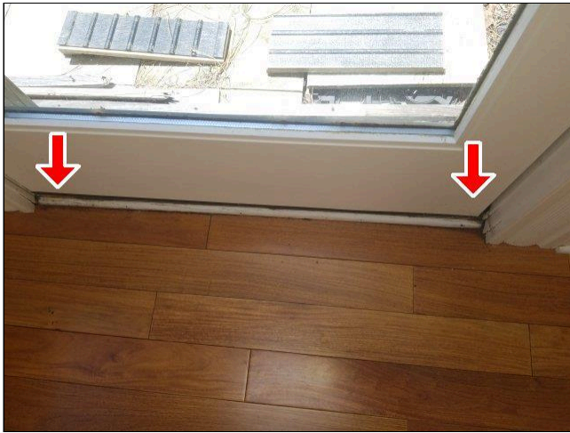
2.2(1) ENTRY DOORS Photo 3
