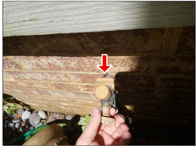
2.11(1) HOSE BIBS / PLUMBING Photo 3
