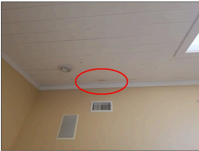
6.6.C(2) WALLS / CEILINGS Photo 1
