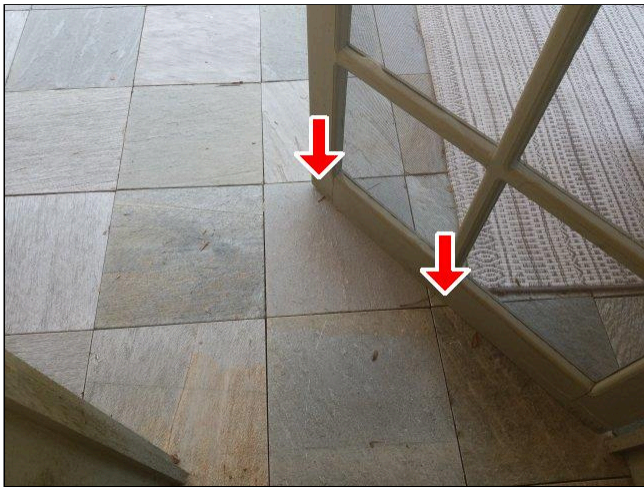
2.2(5) ENTRY DOORS Photo 1
