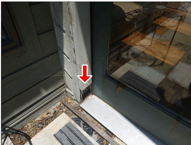
2.2(1) ENTRY DOORS Photo 1
