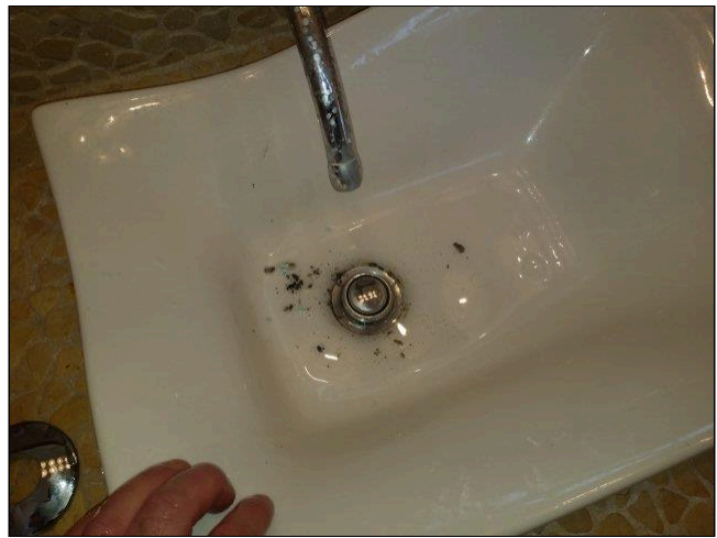
6.0.C SINK(S) Photo 2
