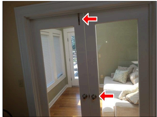
8.7(2) ROOM DOORS Photo 1
