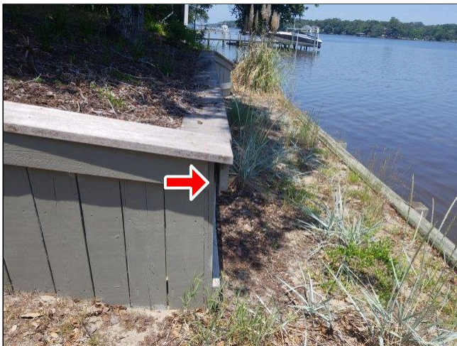
3.2 RETAINING WALL(S) Photo 2
