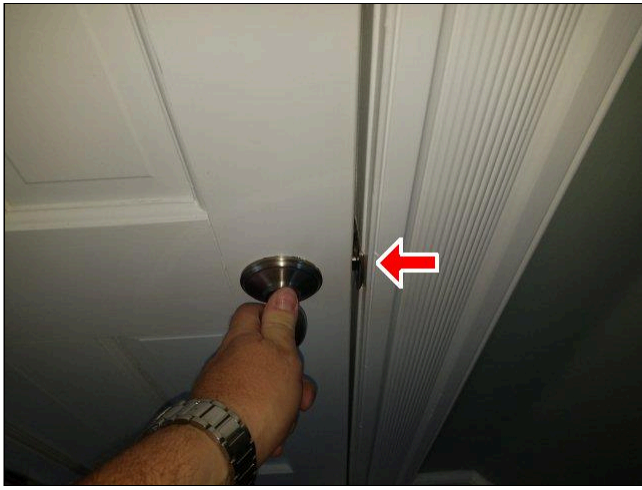
6.5.D WALLS / CEILINGS Photo 1
