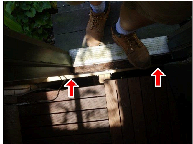
2.2(6) ENTRY DOORS Photo 1
