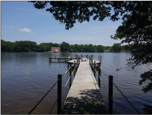
3.5 BULKHEAD / DOCK Photo 1
