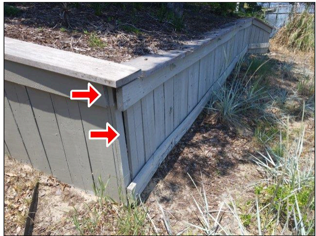
3.2 RETAINING WALL(S) Photo 1
