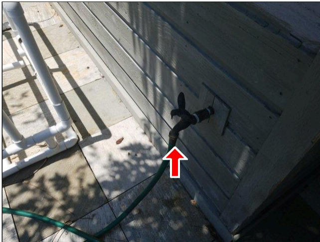
2.11(2) HOSE BIBS / PLUMBING Photo 1
