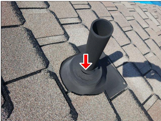
1.6 PLUMBING STACKS Photo 1
