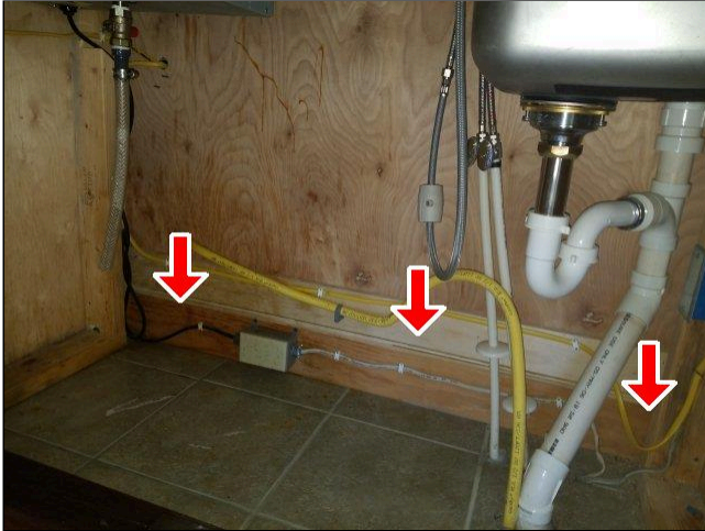
7.3 ELECTRIC / GFCI Photo 1
