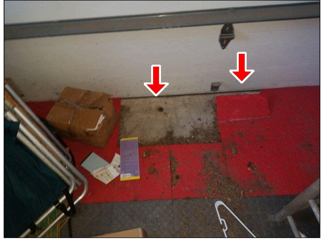
4.3.A FLOOR SLAB Photo 1
