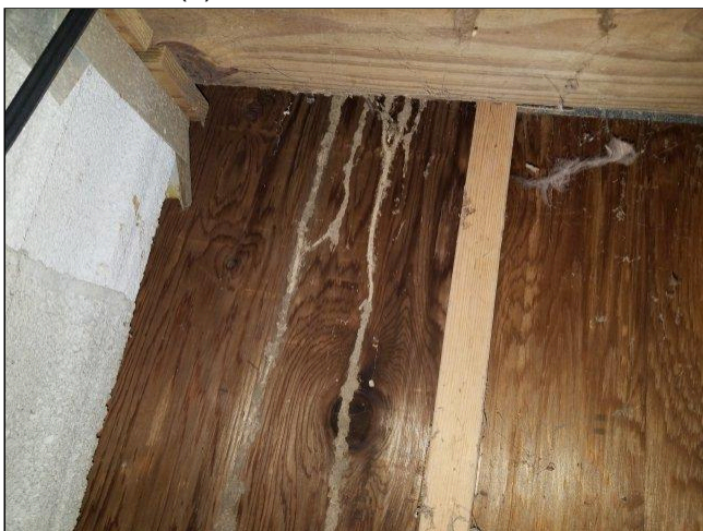
9.2(1) FLOOR FRAMING Photo 3
