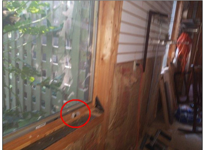
4.5.A WINDOWS Photo 2
