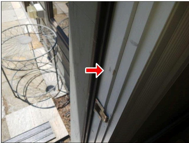
2.2(1) ENTRY DOORS Photo 5
