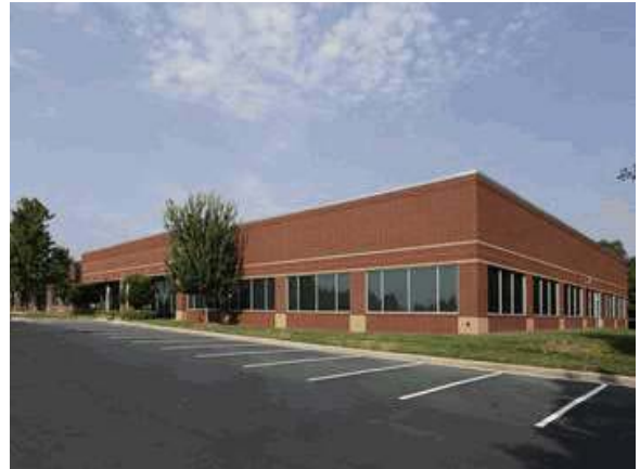
Sale 2 Great Oaks Datacenter
