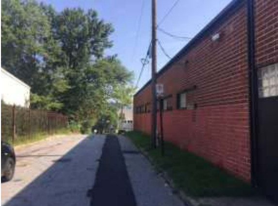
Looking northerly on Curran Street on west-side of Bldg. (Photo Taken on July 20, 2017)
