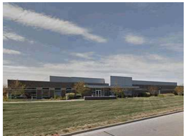
Sale 6 Milwaukee Data Center
