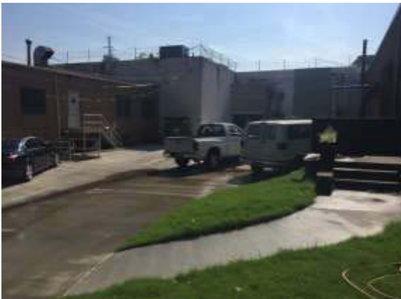
Parking, 48' truck bay and forklift ramp north of Bldg. (Photo Taken on July 20, 2017)
