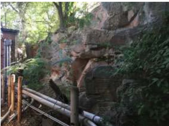
Rear of the building (east-side) (Photo Taken on July 20, 2017)
