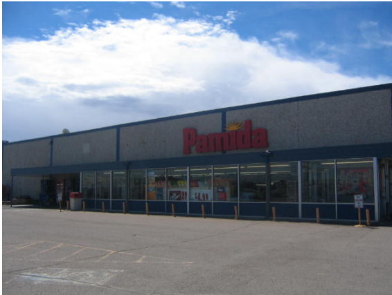
Photo #1: View of the northern elevation of Project
