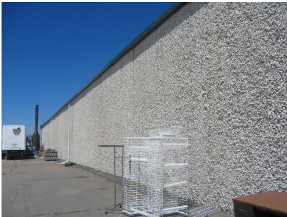
Photo #3: View of the southern elevation of Project
