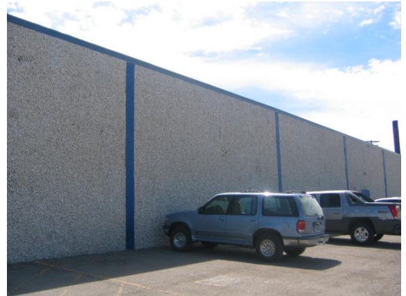
Photo #2: View of the western elevation of Project
