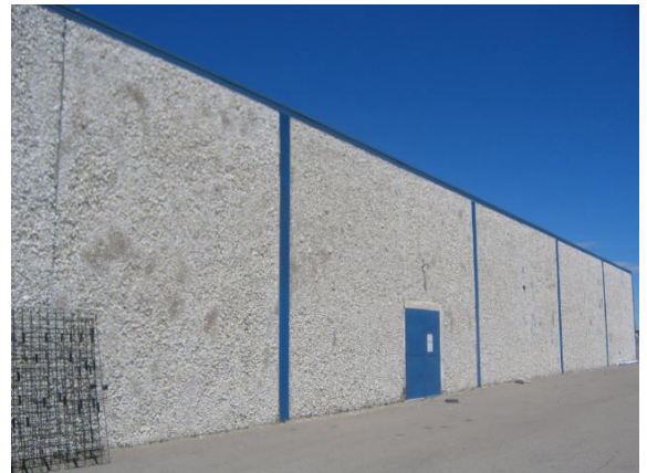
Photo #4: View of eastern elevation of Project
