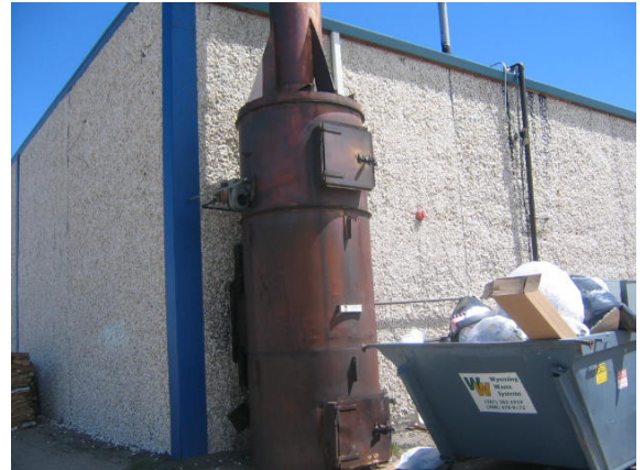
Photo #8: Non-operational cardboard incinerator located on the southwest corner of Project building
