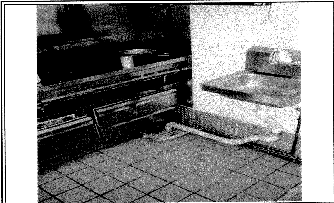
Photograph depicts floor drain located inside kitchen area of site building.
