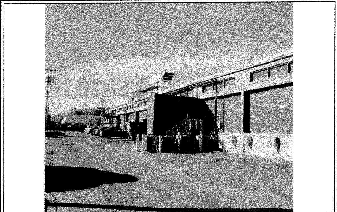
Photograph depicts south side of the site building.
