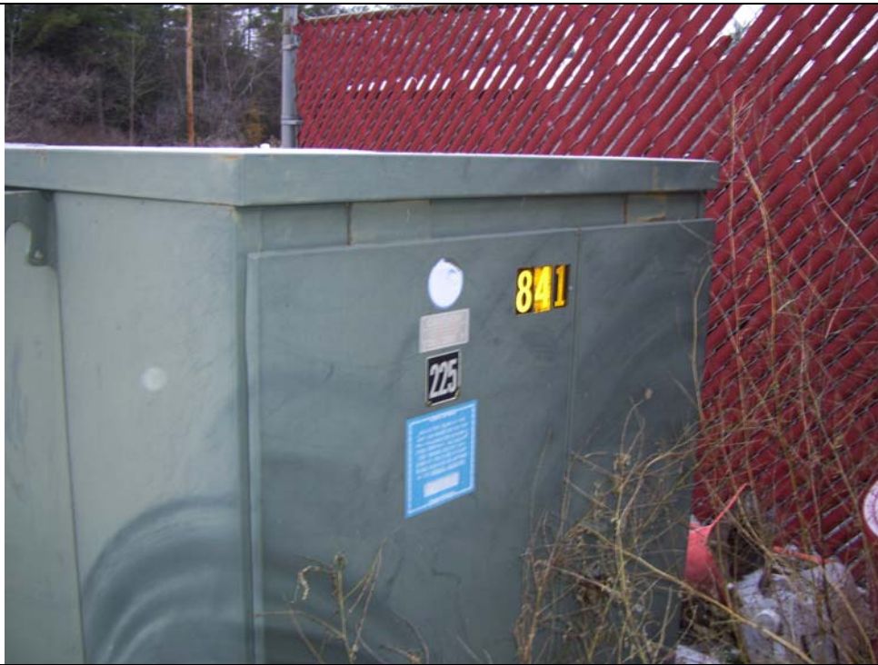
PHOTOGRAPH DEPICTS VIEW OF PAD MOUNTED TRANSFORMER.
