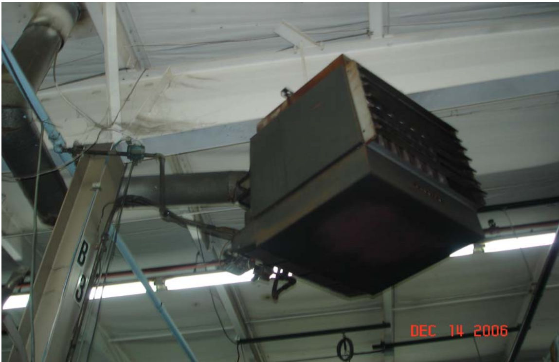
View of the space heaters (gas fired).
