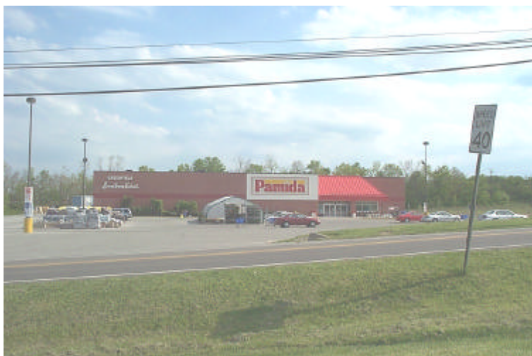
Facing south across Jefferson Street with an overview of the subject.
