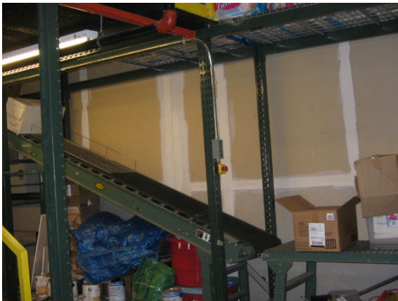
Photo #9: Electronic conveyor belt to mezzanine level in storage room
