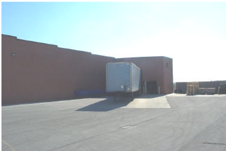
View of the shipping/receiving area
