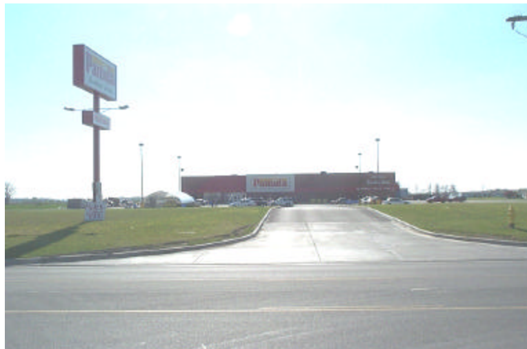
Facing west across South Defiance Street with an overview of the subject.
