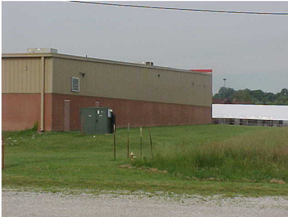
Photo #1: North side of Project
