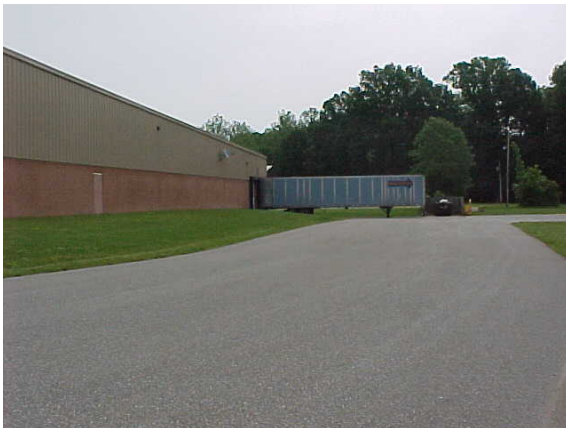
Photo #3: South side of Project
