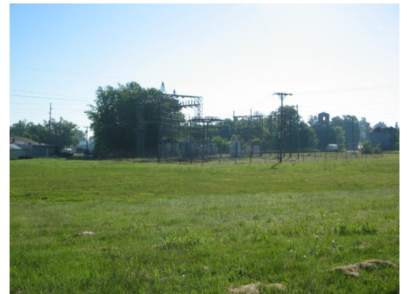
Photo #18: Adjacent east — electrical substation
