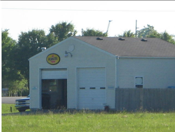
Photo #19: Adjacent east — Vic's Service Center
