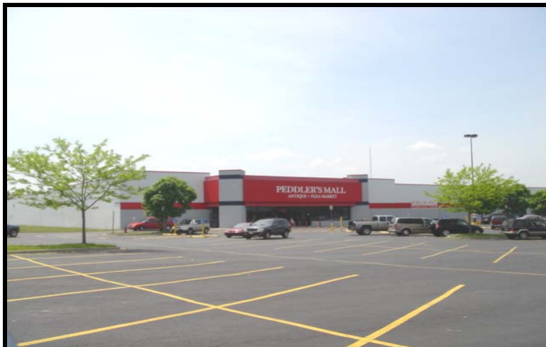
Comparable 3 – Former Wal-Mart building, Georgetown, KY
