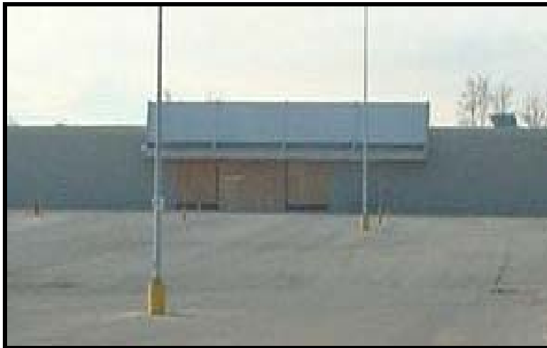
Comparable 2 – Former K-Mart building, Louisville, KY
