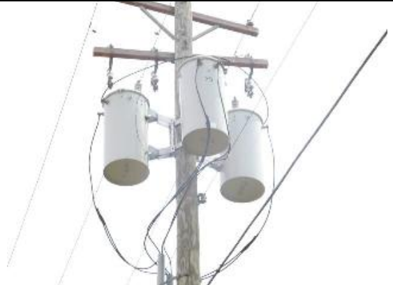
Photo #10: Pole mounted transformers. Section 5.1
