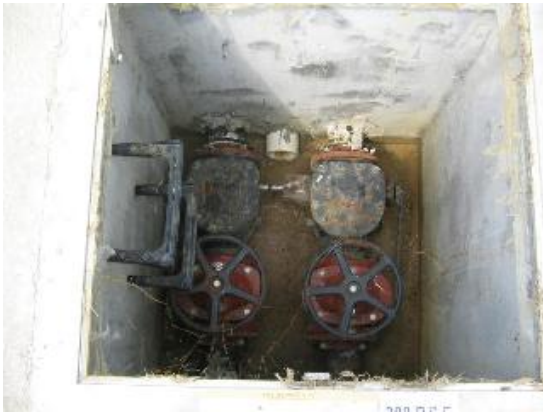
Photo #7: Water vault. Section 5.1
