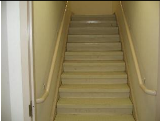
Photo #29: Interior stair. Section 6.5
