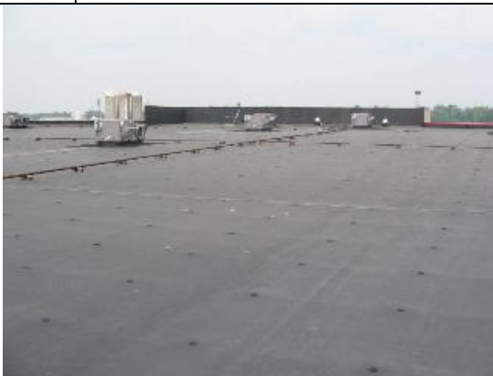
Photo #5: Roof overview. Section 6.3
