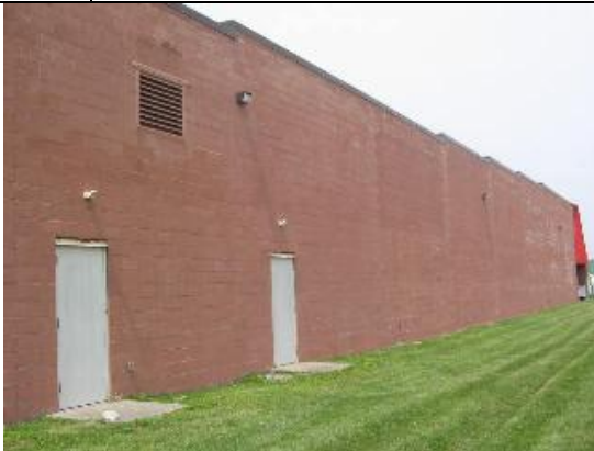
Photo #3: North elevation of building. Section 6.4
