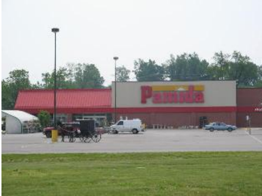
Photo #1: Front elevation of building. Section 6.4
