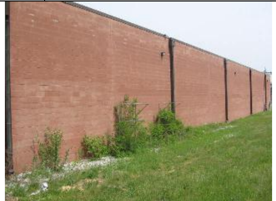
Photo #4: Rear elevation of building. Section 6.4
