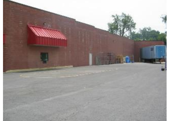
Photo #2: South elevation of building. Section 6.4
