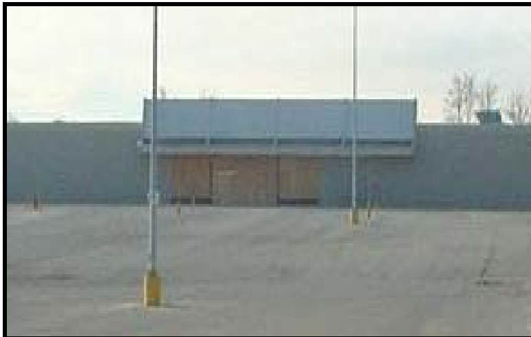
Comparable 2 – Former K-Mart building, Louisville, KY
