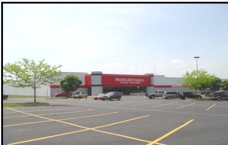
Comparable 3 – Former Wal-Mart building, Georgetown, KY
