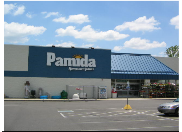
Photo #2: Front of building
