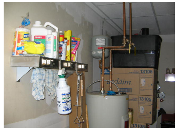
Photo #12: Janitor's supplies and water heater
