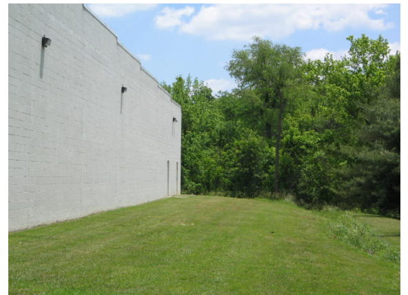
Photo #6: West side of the Project looking to the south
