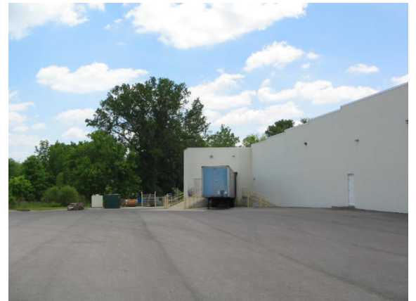
Photo #4: East side of the Project, looking to the south
