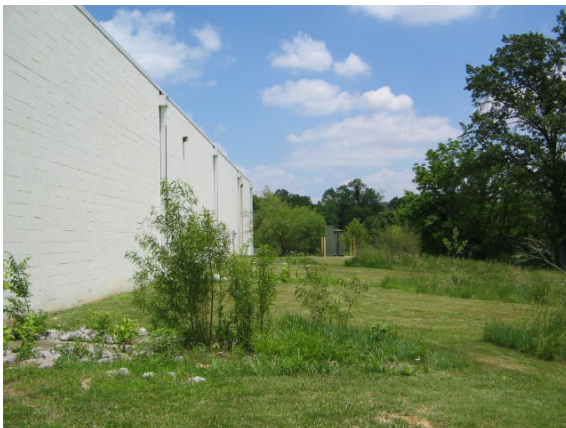
Photo #5: South side of the Project, looking to the east
