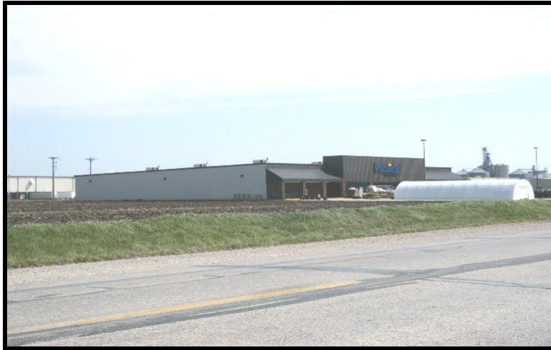
04 – Exterior view of the southwest corner of the subject
