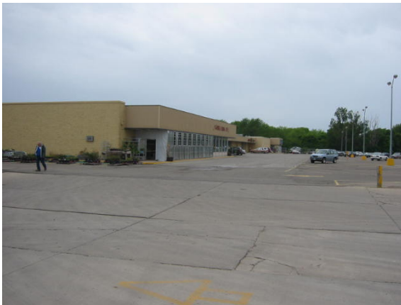
Photo #15: Property adjacent to the west — Alco Discount Store, no issues
