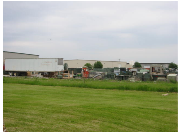
Photo #16: Property adjacent to the south — Western Power Electra Mold Company, no issues
