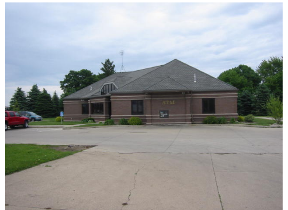
Photo #18: Property adjacent to the east — Credit Union, no issues
