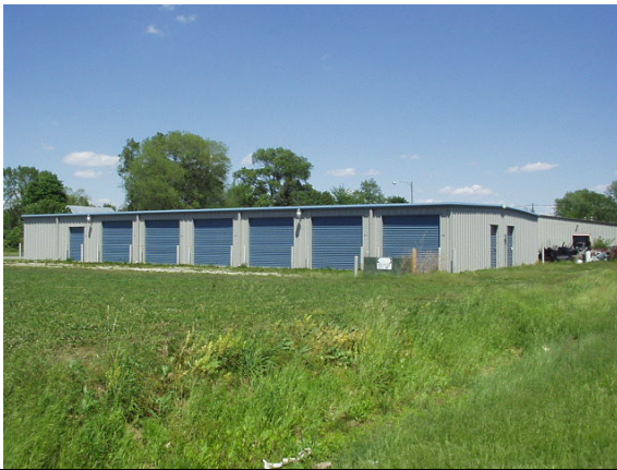
Photo #15: Adjacent property north — mini-storage facility
