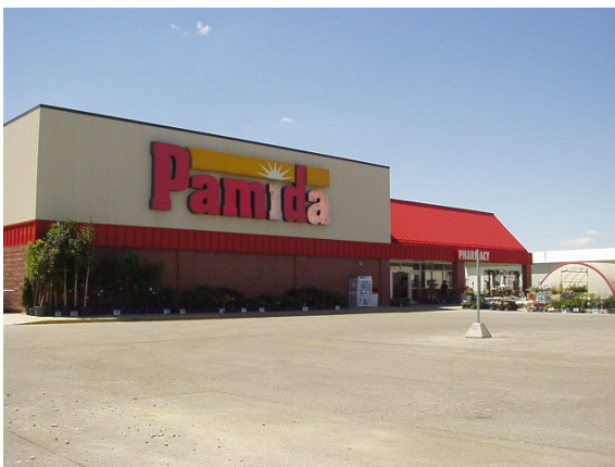
Photo #5: Front entrance to building
