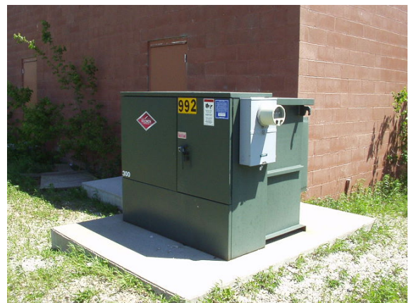
Photo #6: Transformer installation
