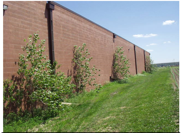
Photo #2: Rear elevation of building
