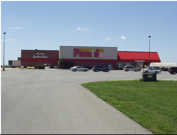
Photo #1: Front elevation of building
